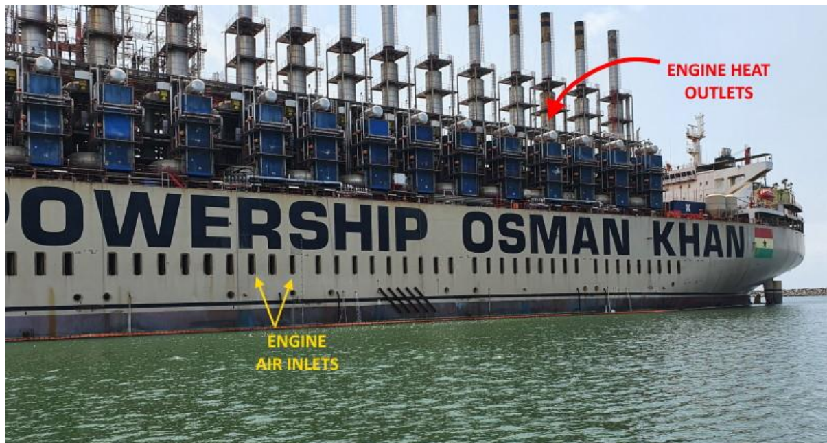
Figure 3-1 Powership photograph showing the primary noise sources
