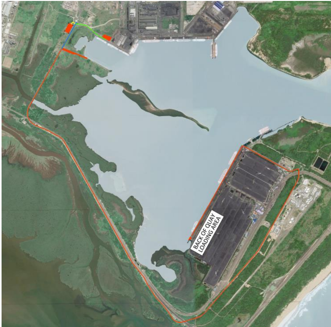
Figure 5: Back of Quay Loading Area (Source: PRDW S2117-07-DR-GA-202-S1-A)
