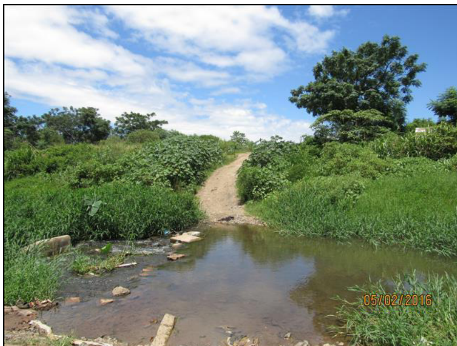
Plate 1. A view of the proposed location for Tottenham Road Pedestrian Bridge.
