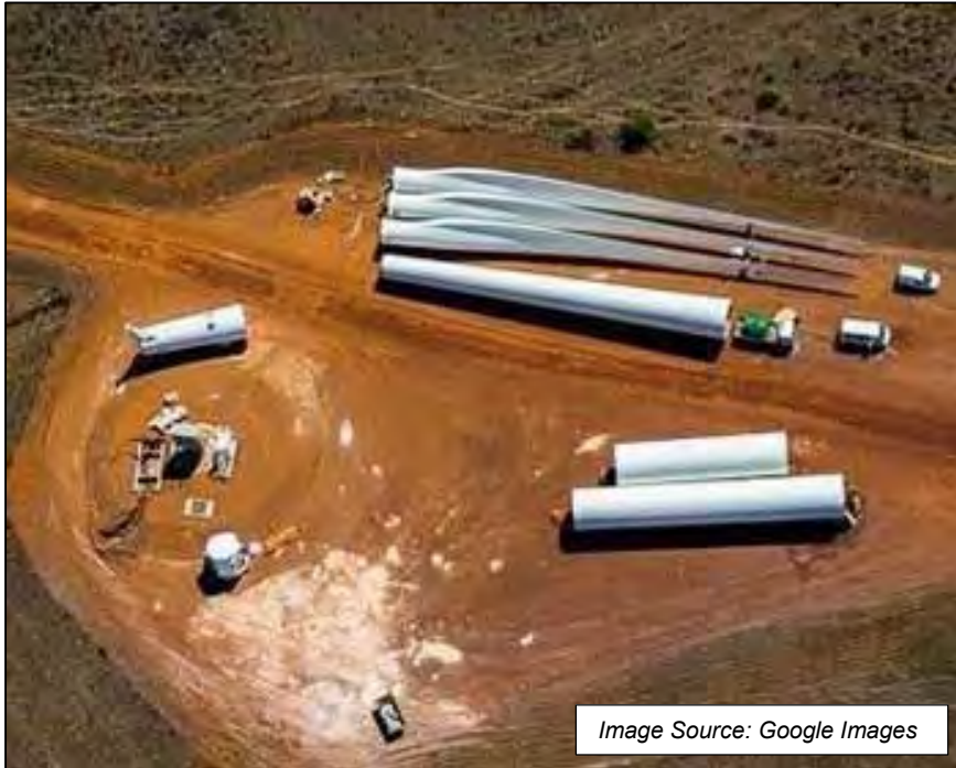
Figure 4.2 - Typical Laydown area for Turbine Components
