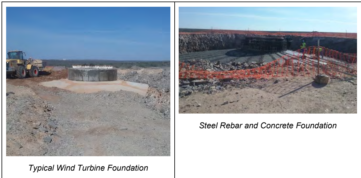
Figure 8.1 – Concrete Foundations
