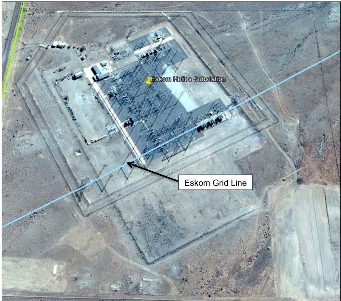
Figure 10.6 - Helios Substation Location
