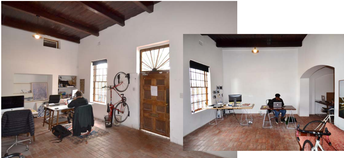
Office space. Original spaces with 3,8m high ceilings (c 1850's). Brick floor, bead mould ceiling beams, modern pine ceiling boards, modern sash windows, modern entrance door and fanlight, modern flat arched openings between rooms (c 1970/80).
