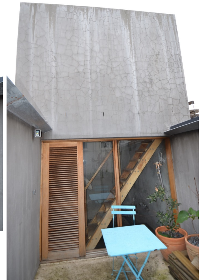
Mezzanine court space. Modern Poplar door with shutter and fixed full height side panels, modern Poplar open stair access to roof deck, modern special galvanised gutters (c 2013/14).
