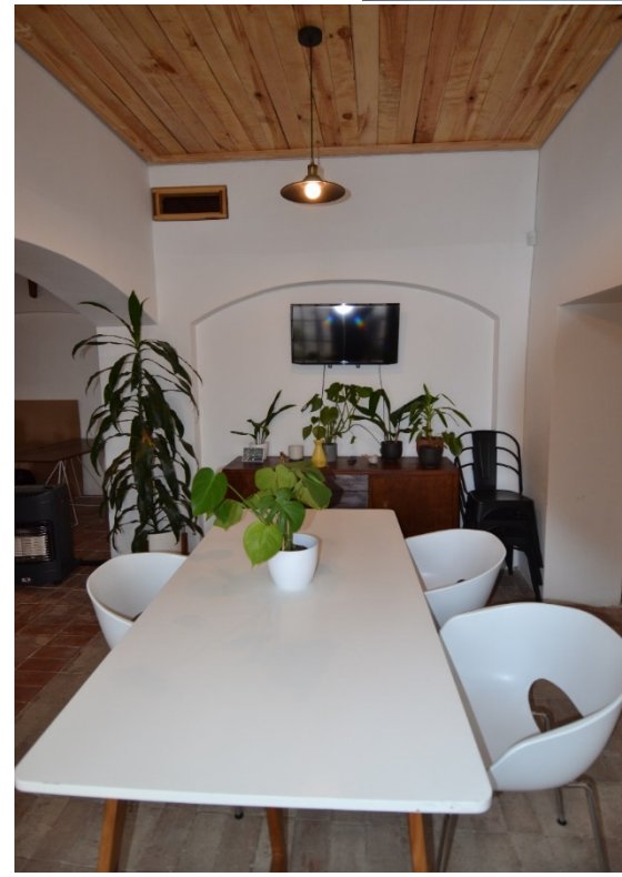
Office space. Brick floor, modern pine ceiling boards, modern double doors, modern flat arched openings between rooms (c 1970/80). Modern square high level square window (c 2013/14).
