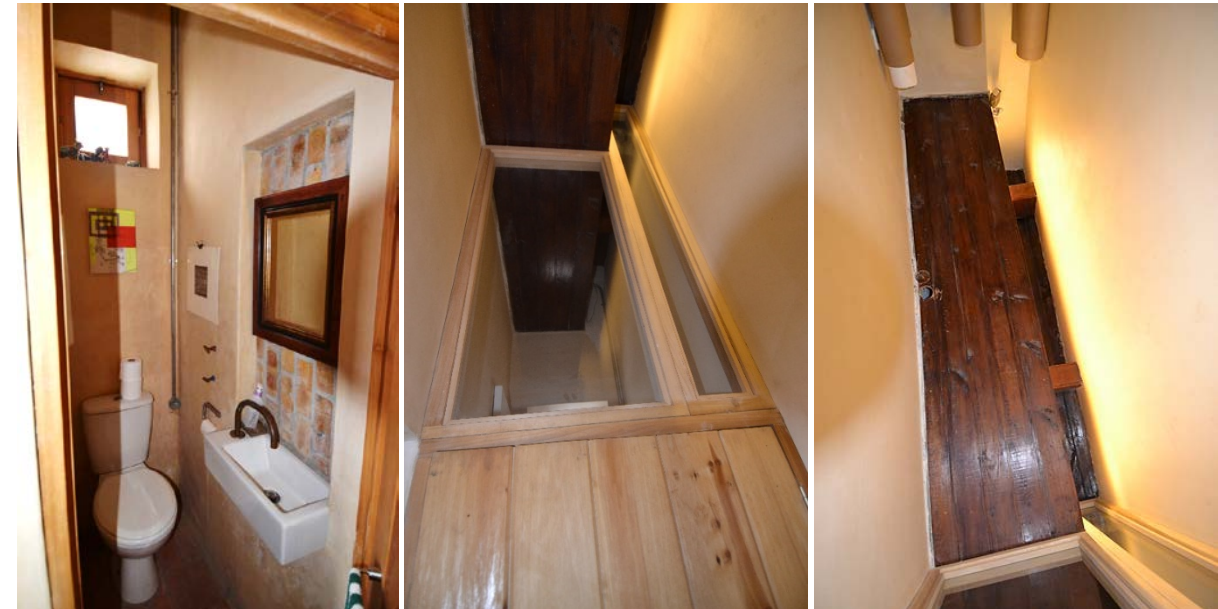
WC off gallery space, modern Poplar door with tall fanlight, high level dropped ceiling storage space, modern sanitary ware, recessed exposed brickwork splashback, square high level windows (c 2013/14).
