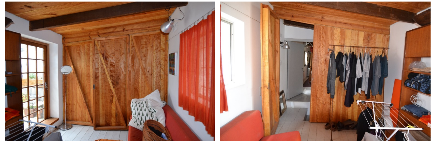
Guest bedroom space. Modern door to court, modern ceiling beams and ceilings (c 1970/80), modern Poplar vertical slatted and framed timber wall panels with diagonal bracing and integral doors between stair well/guest bedroom and guest bedroom/guest bathroom (c 2013/2014).
