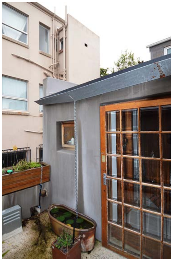
Mezzanine court space. Modern door (c 1970/80), modern special galvanised gutters (c 2013/14).
