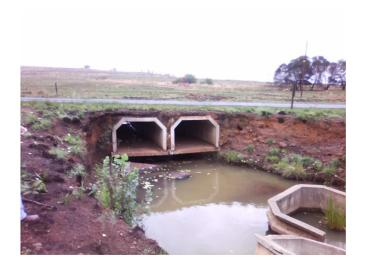
The culvert has already lost some of its spans, together with the outlet structure.
