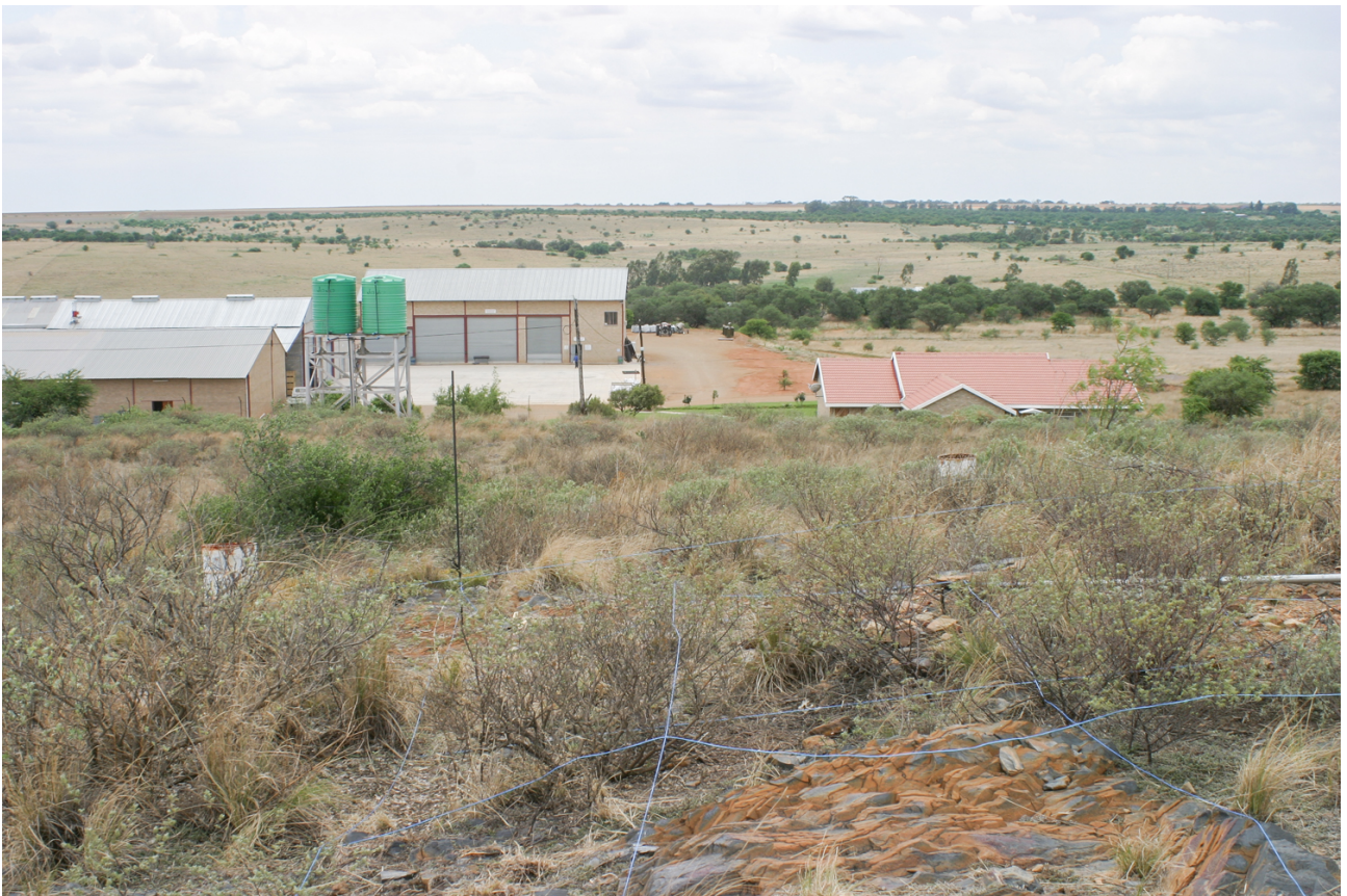
Figure 12. Looking eastwards from the rock art site on top of Gestoptefontein Hill: the main plant (left) and offices (right).
