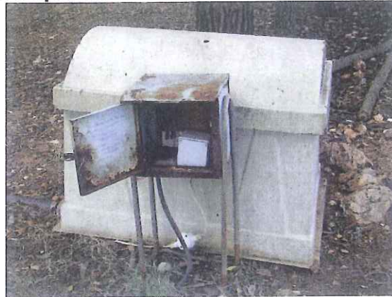
Groundwater abstraction from a borehole
