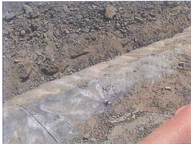
Hazardous waste disposal facility with HDPE liner
