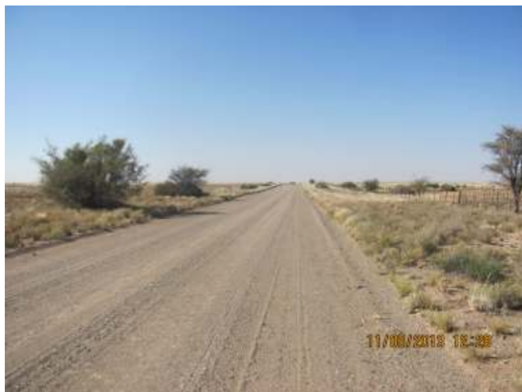
Figure 2: Showing District Road D3276
