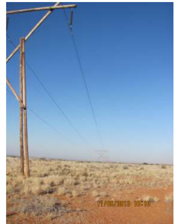
Figure 9: Existing 133Kv Powerline on the adjacent property.
