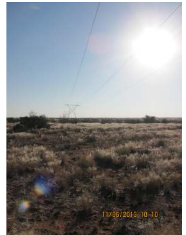
Figure 10: Existing 133Kv Powerline crossing the property.
