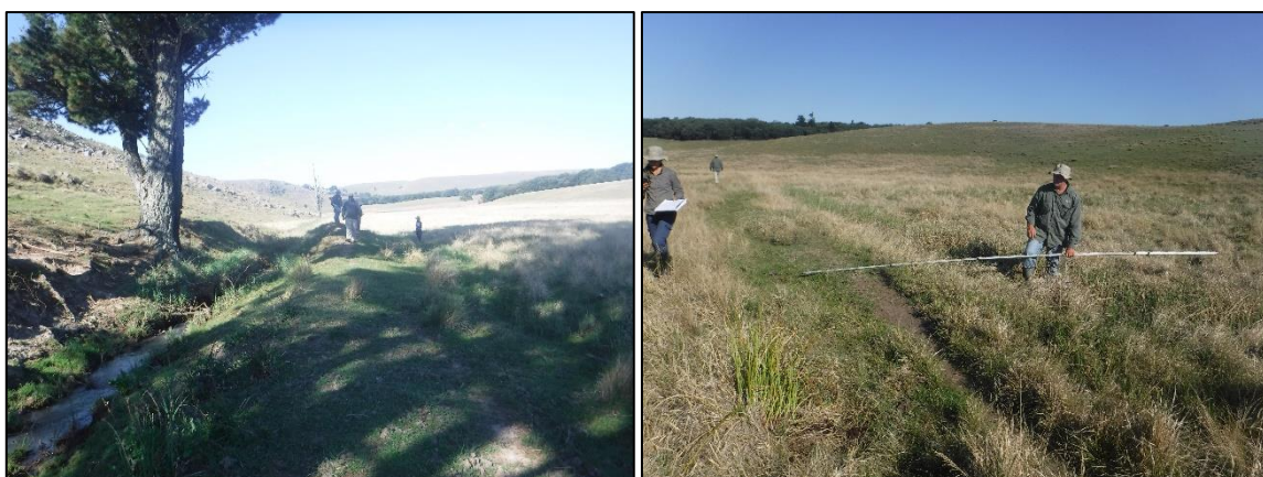
Figure 4.6 The straightened channel running down the left-hand bank of the wetland (left), and a berm limiting diffuse flows through the wetland (right)
