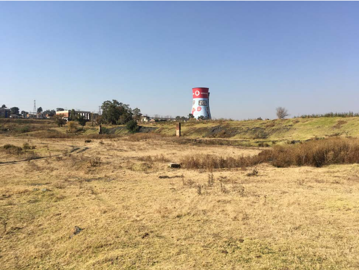
17. Conveyor columns for ash delivery downstream of the embankment
