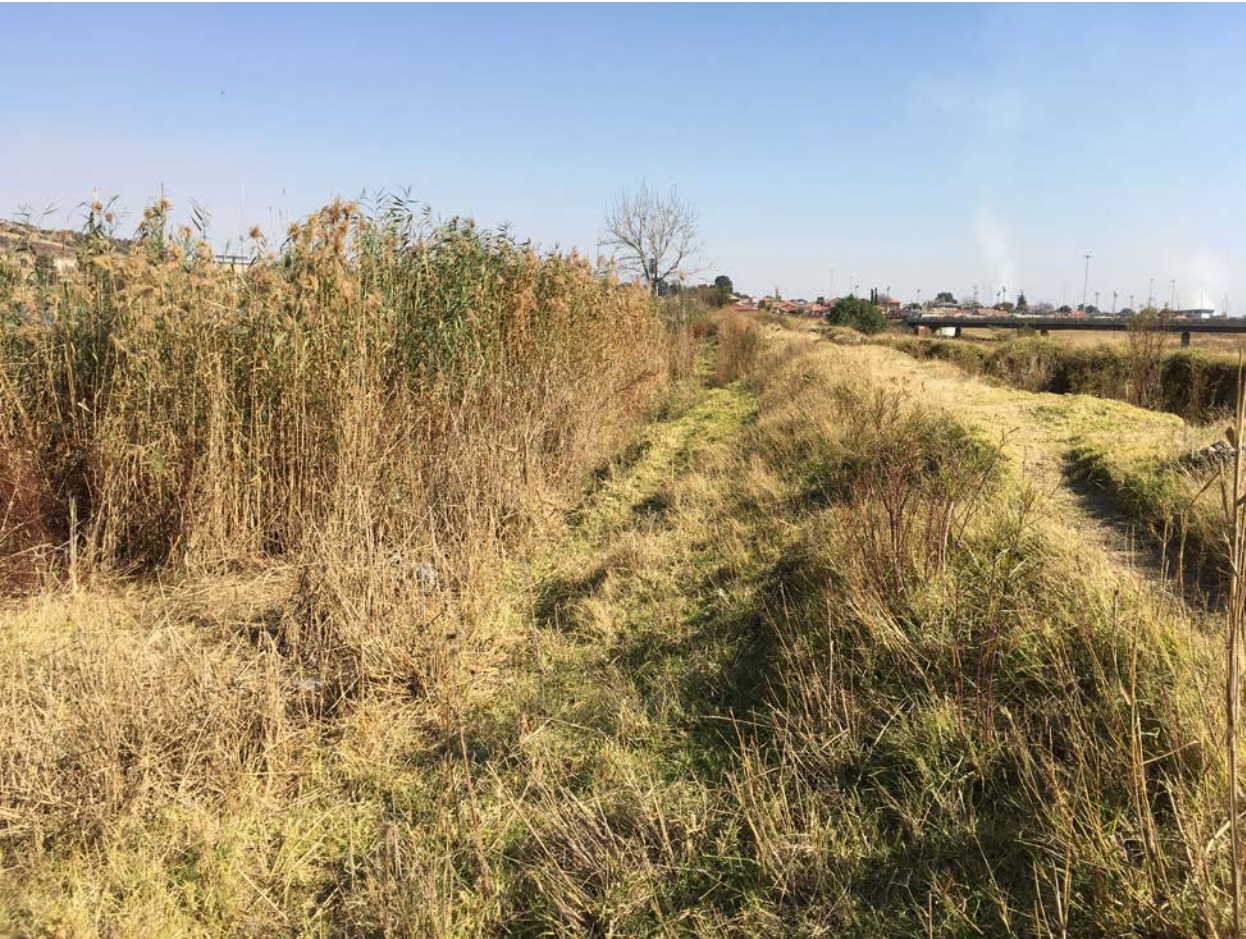
9. Poor condition of the NOC illustrating lack of maintenance.
