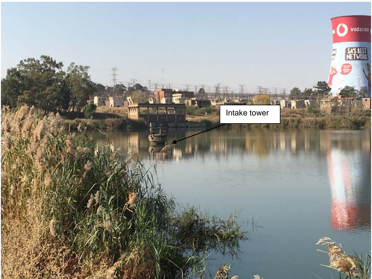
8. View of the intake tower, NOTE the dense reeds surrounding the embankment
