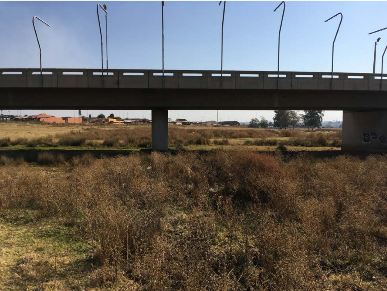
18. View of heroes bridge downstream of the Embankment.
