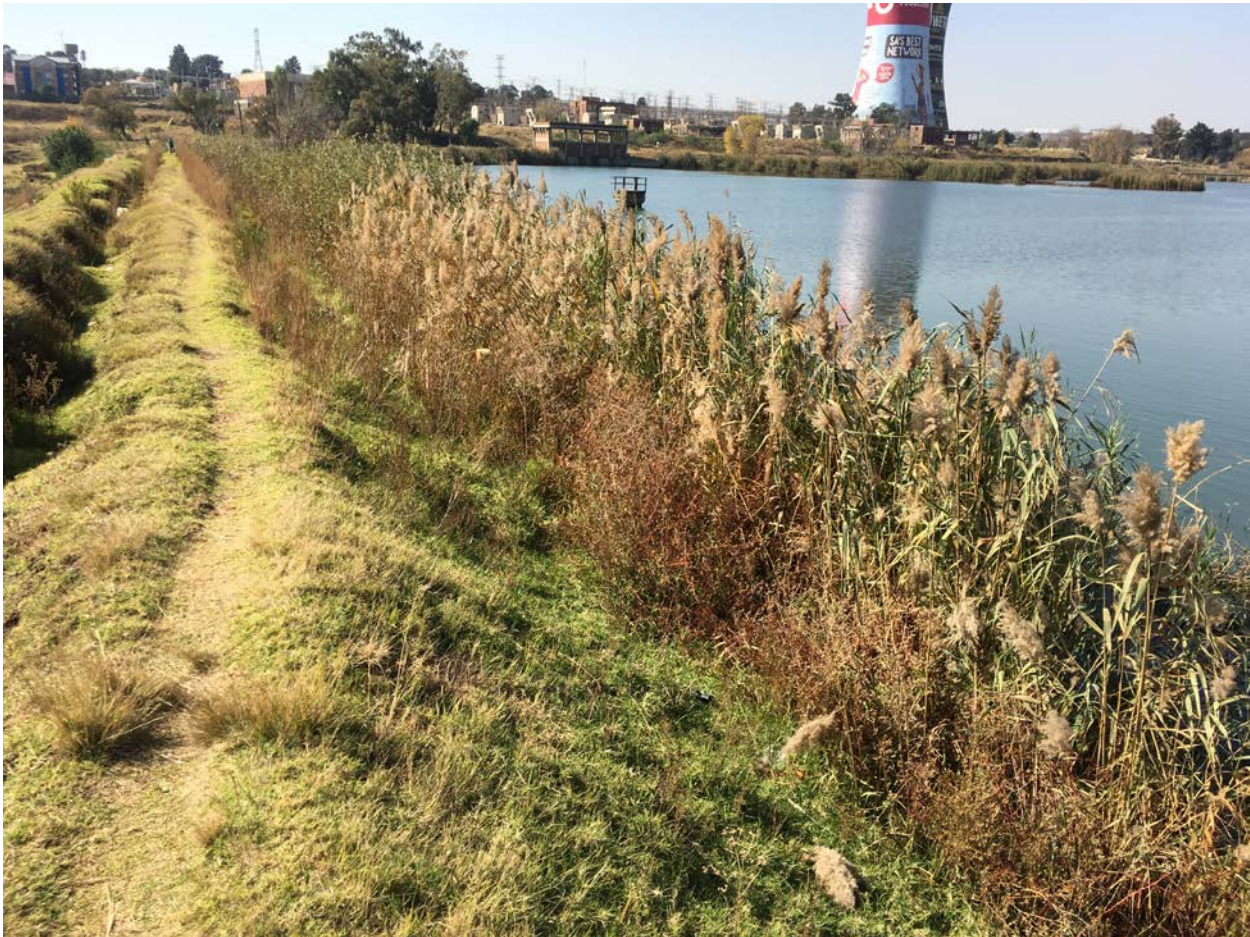
5. Reeds on the upstream slopes (routine maintenance required)
