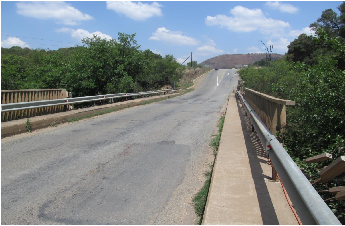
Photo 7: Bridge 649 over the Hennops river towards the South
