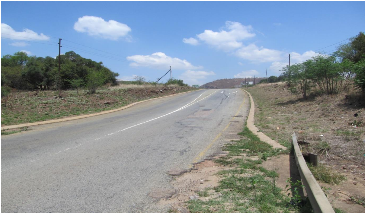
Photo 1: Road P246 towards the South East
