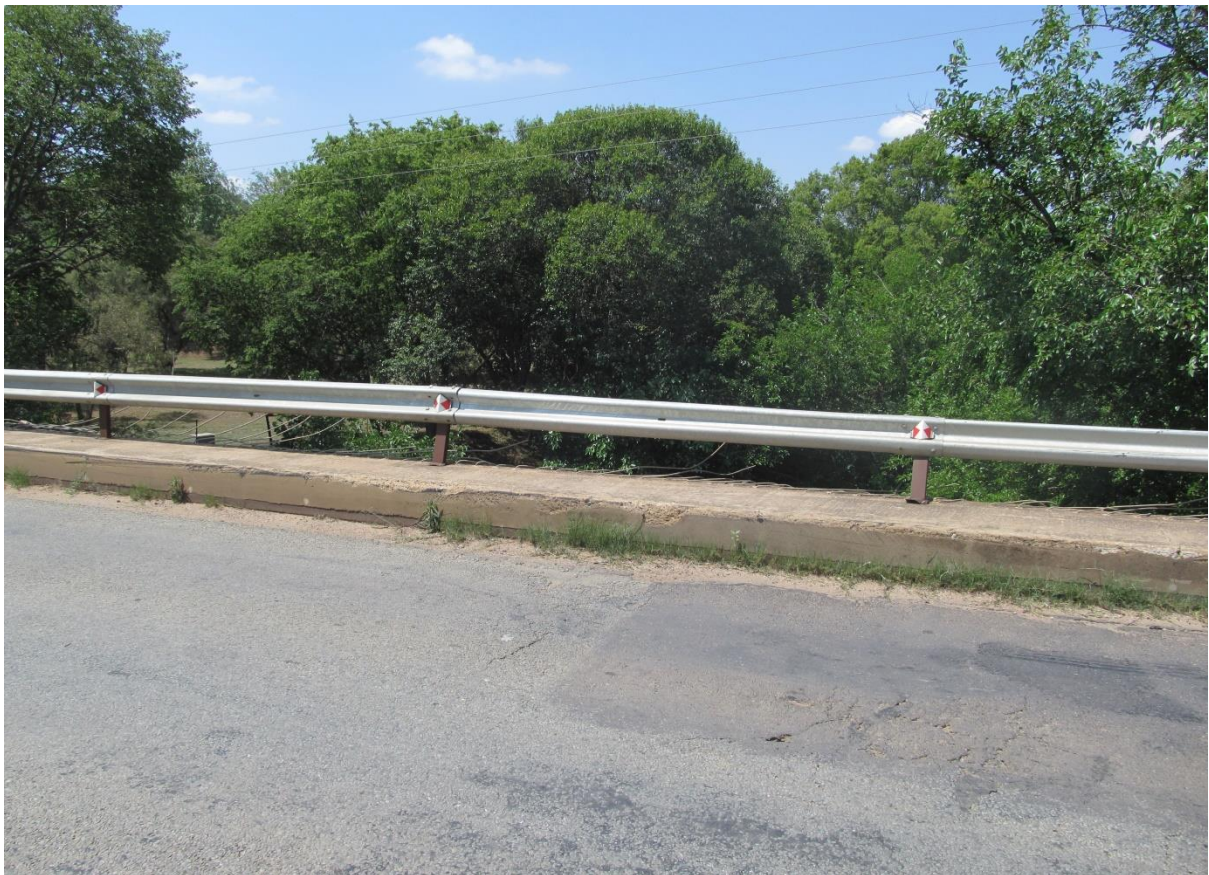
Photo 6: Bridge 649 over the Hennops river towards the East
