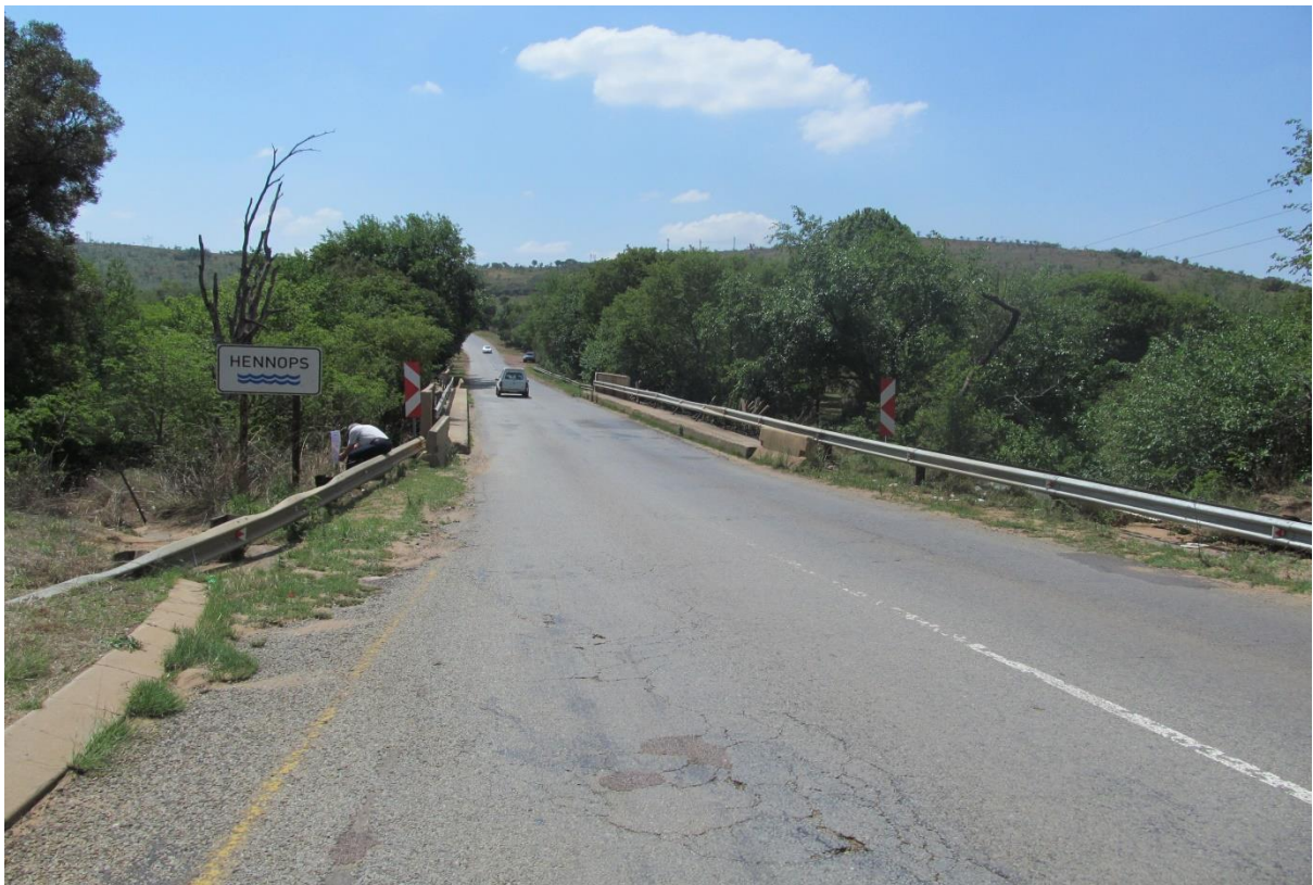
Photo 2: Bridge 649 over Hennops river towards the North West
