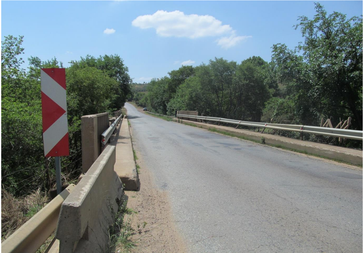
Photo 4: Bridge 649 over Hennops river towards the North
