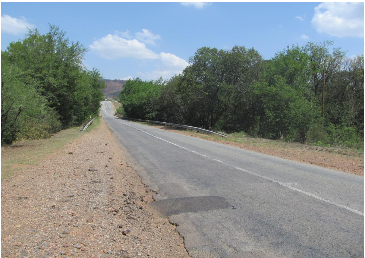
Photo 12: Road P249 and Bridge 649 towards the South West
