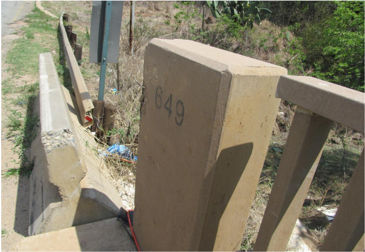
Photo 3: Bridge 649 over the Hennops river towards the West
