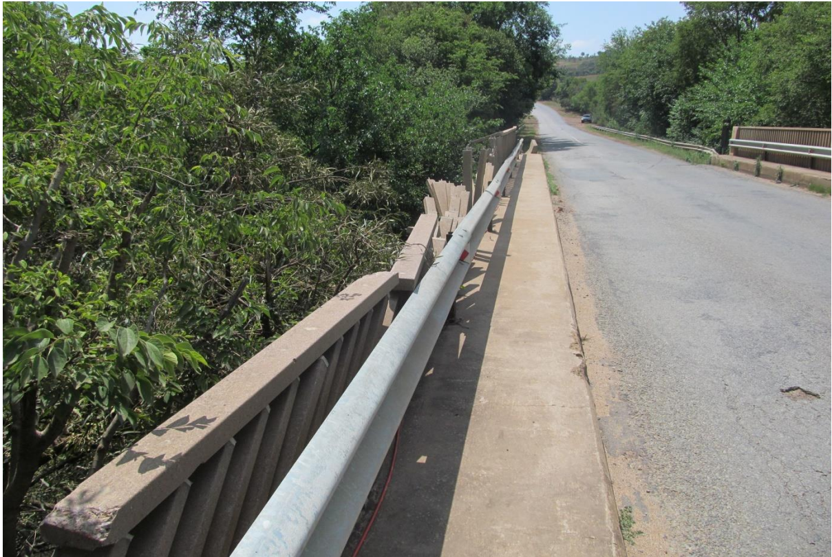
Photo 5: Bridge 649 over Hennops river towards the North East
