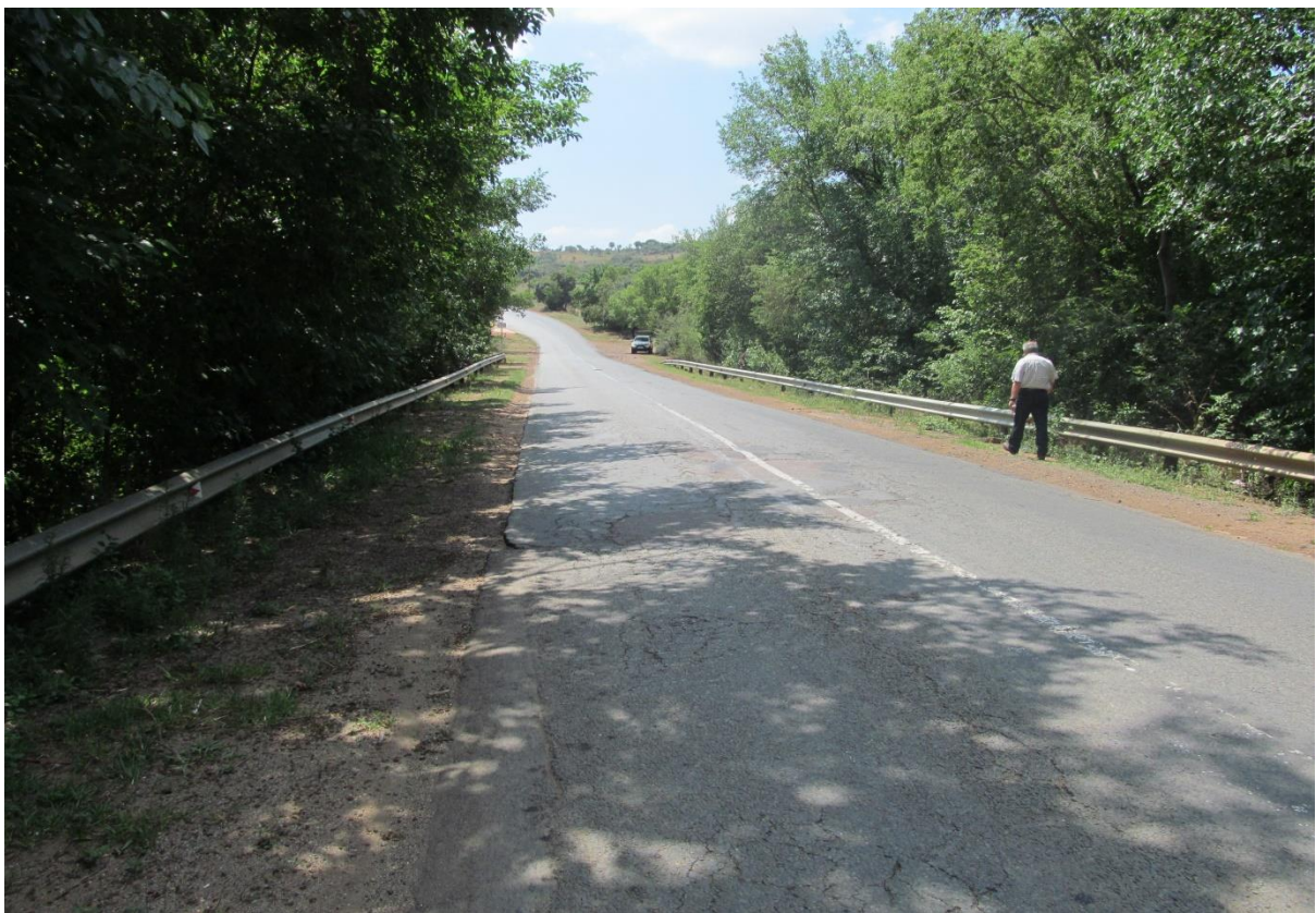
Photo 8: Road P249 towards the North West
