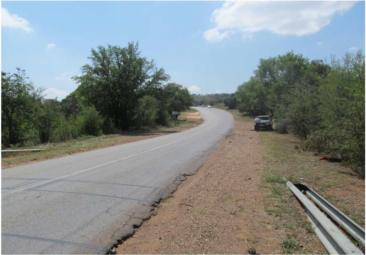
Photo 11: Road P249 towards the North West
