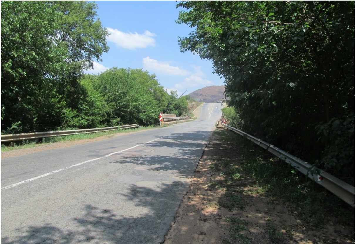
Photo 9: Bridge 649 over the Hennops River towards the South East
