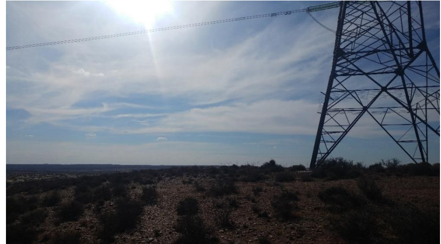
Existing Powerline north of the proposed Dwarsrug Access Road Access road
