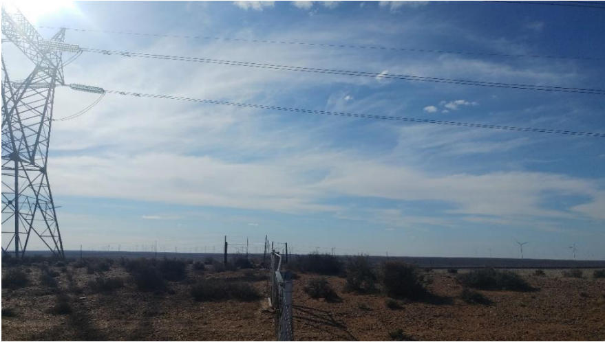
Existing Powerline north of the proposed Dwarsrug Access Road
