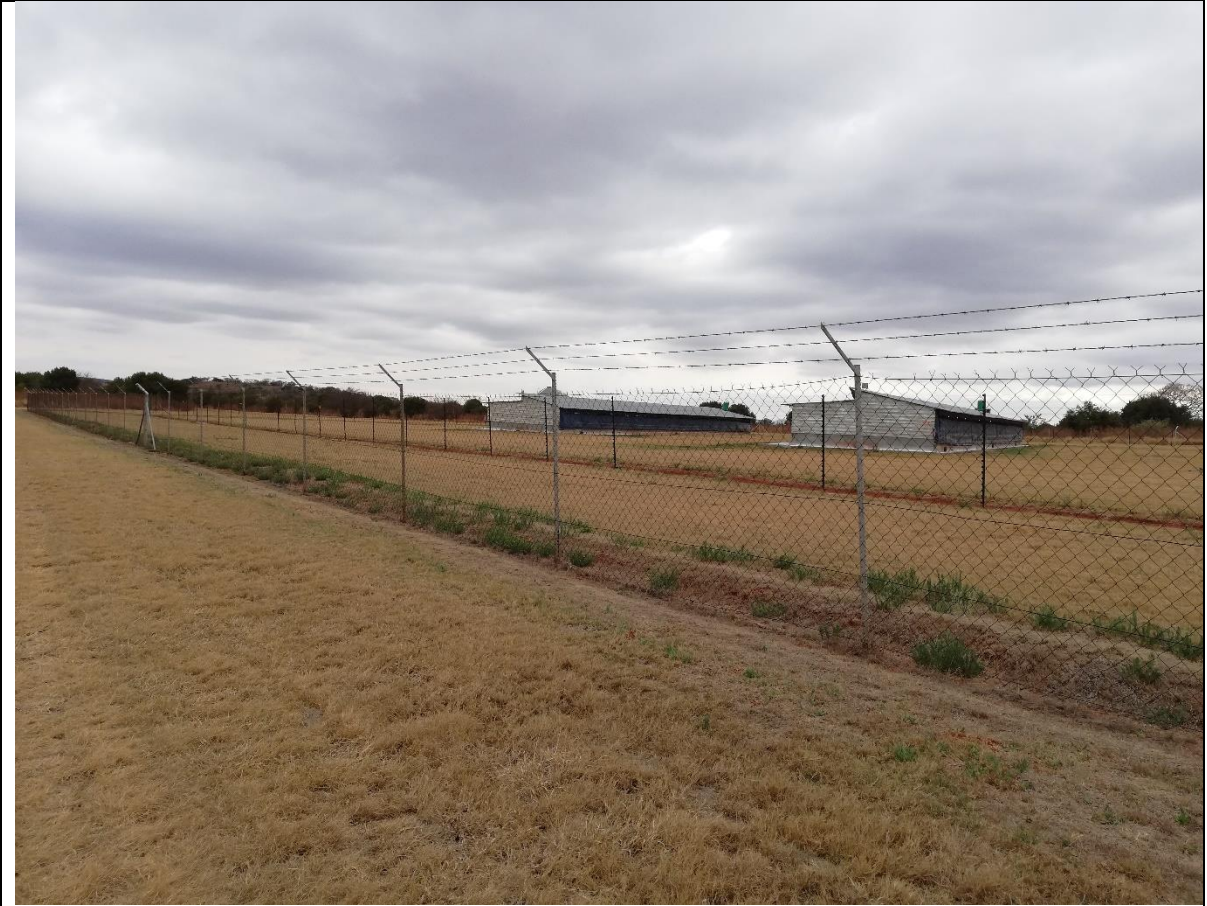
Site 2b (Evaporation Pond and Chicken House Development):
