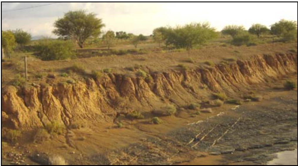
Figure B18: Bridge NB38: View to the downstream of the bridge (facing south-west)
