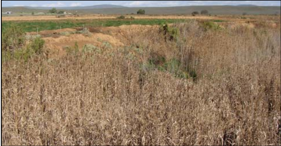
Figure B9: Bridge NB36: View of vegetation upstream of the bridge (facing south)
