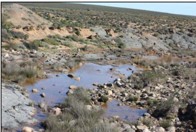
Figure B3: Bridge NB35: View to the downstream of the bridge (facing west)(Photo provided by Aurecon)
