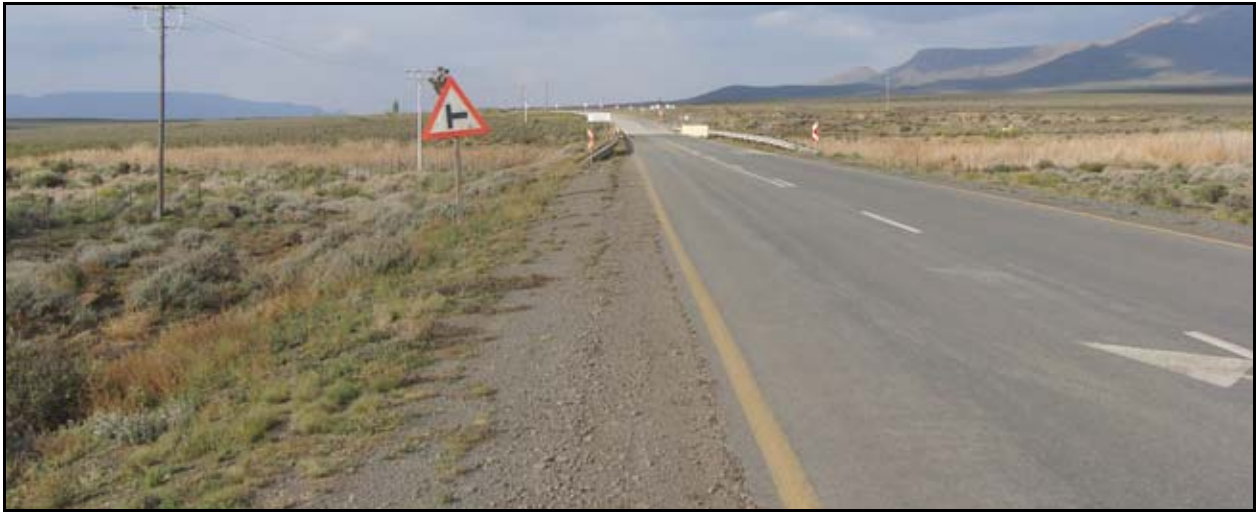
Figure B10: Bridge NB37: View of the R27 across the bridge (facing east)
