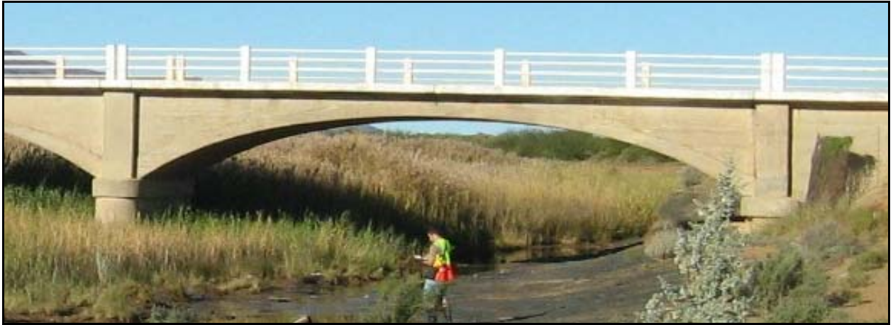
Figure B16: Bridge NB38: View of the bridge from within the watercourse (facing west)(photo provided by Aurecon)
