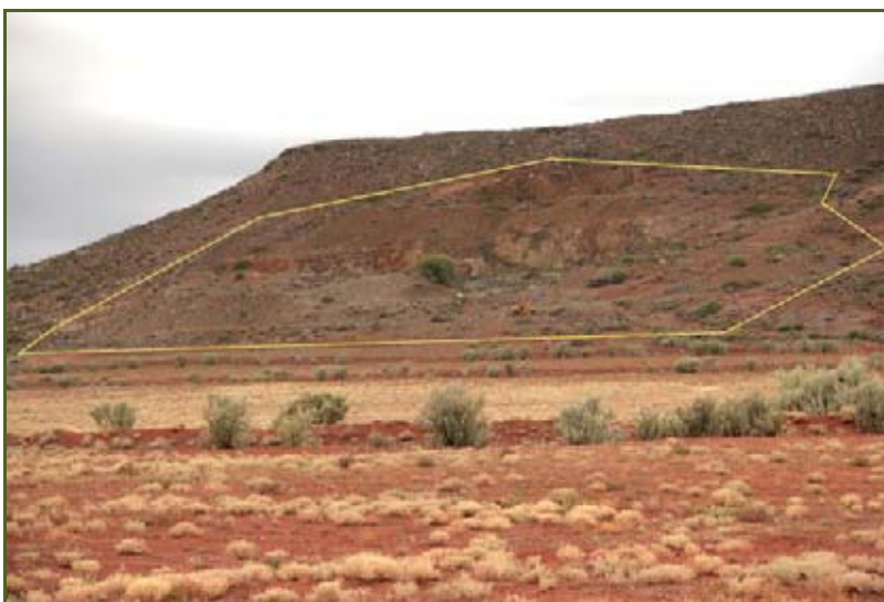
Figure B21: BP R27-8 KM 32.6 RHS 6.2: View of the site, with the abandoned Iceland Spar mine outlined in yellow (facing south-east)(photo provided by Dr D MacDonald)
