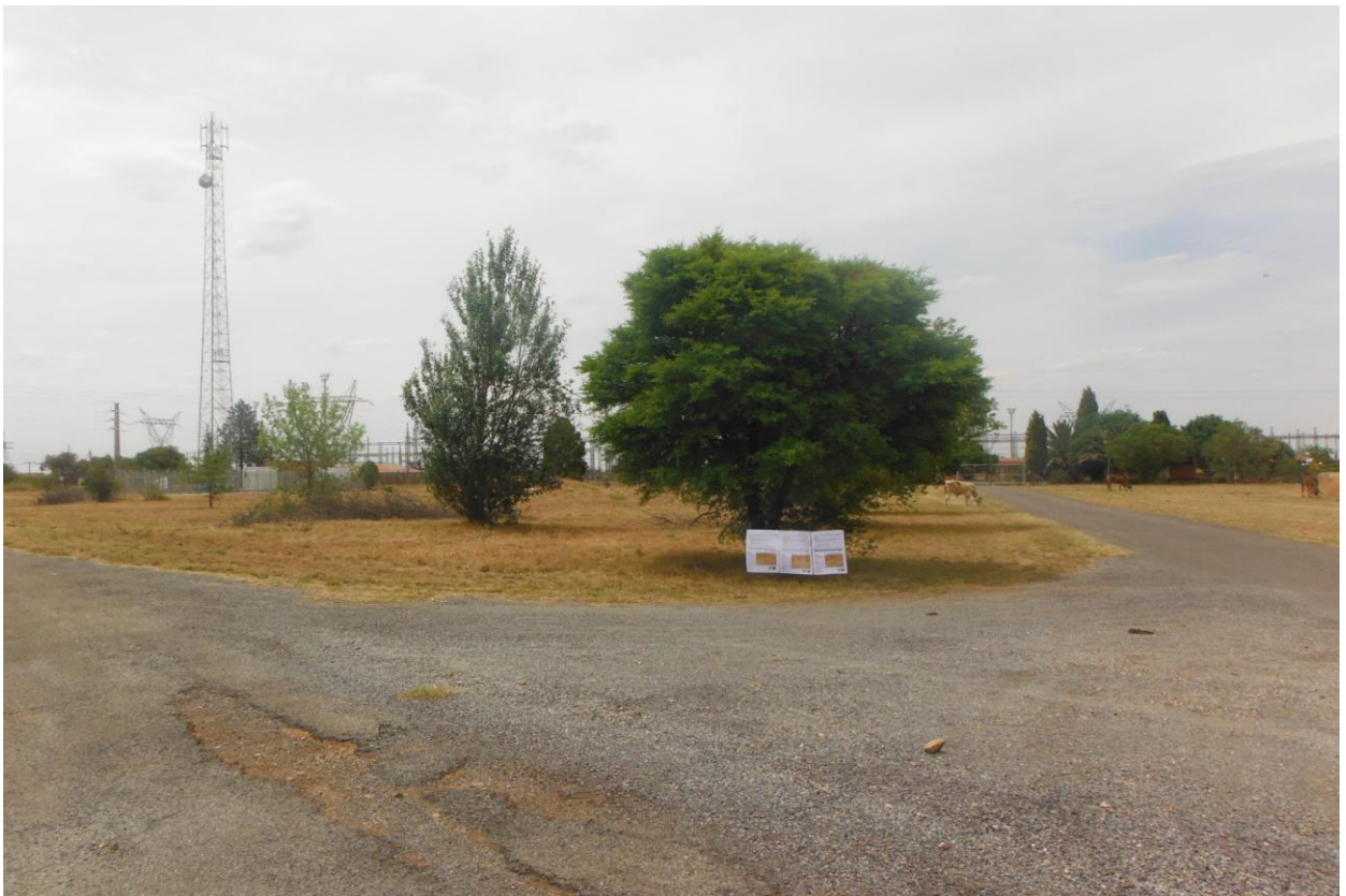
Figure 9: View of the site towards the east of the south of the substation
