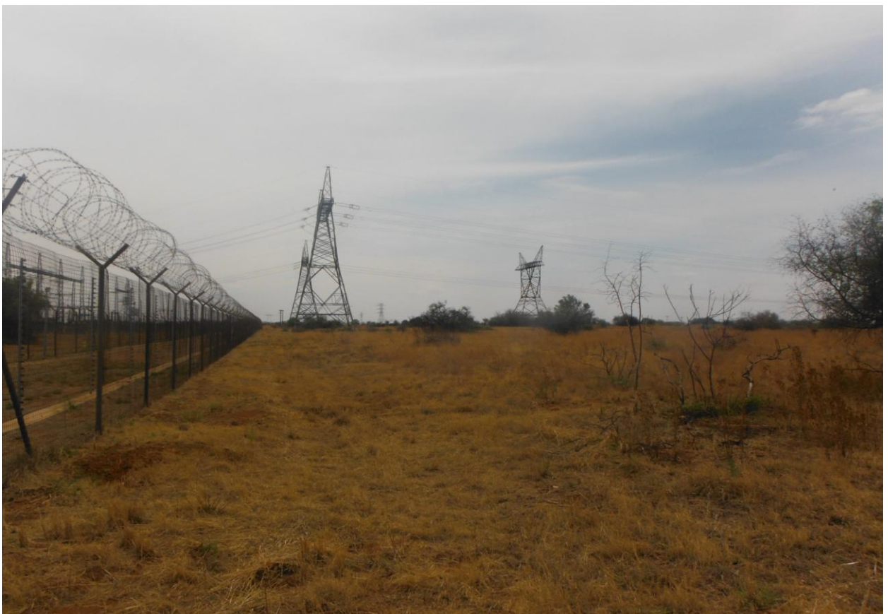
Figure 7: View of the site towards the east of north of the substation
