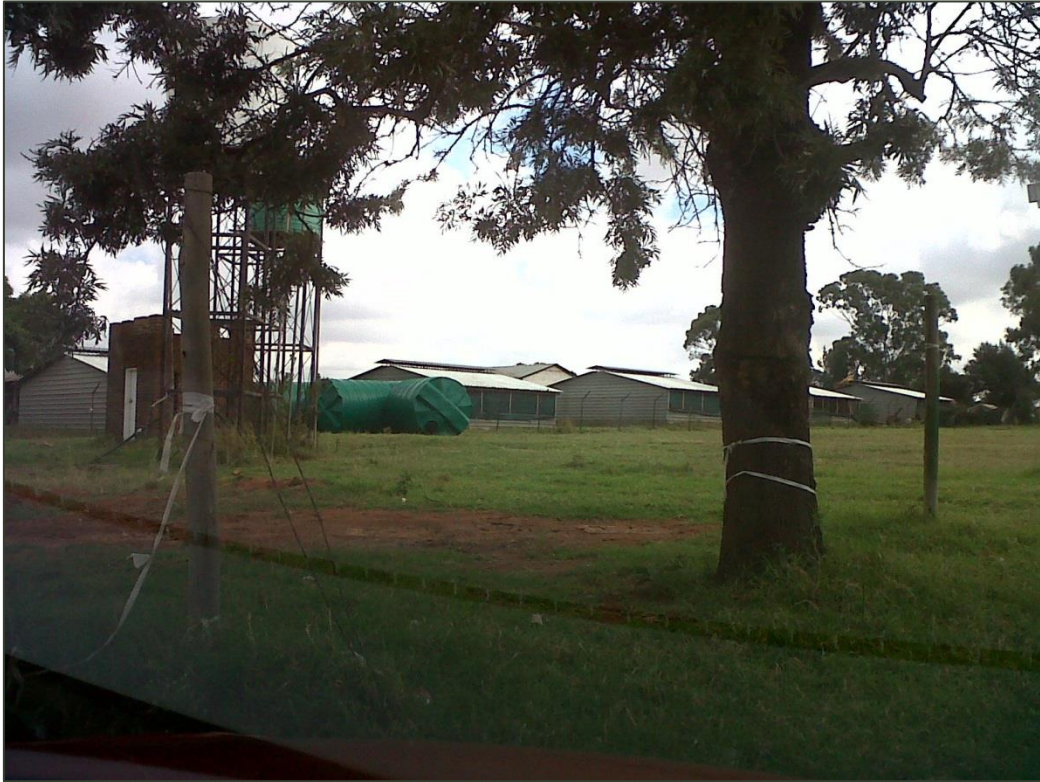
Figure 3: Existing poultry houses
