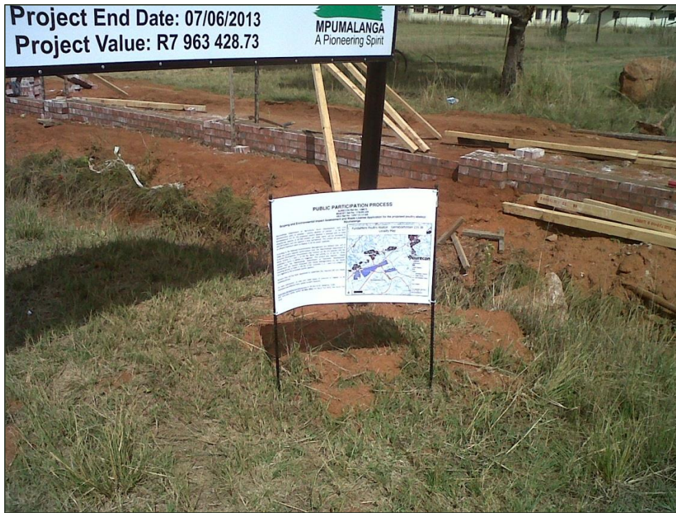
Figure 1: Site notice placed at the entrance to the existing poultry houses
