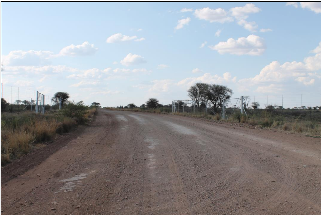
Plate 10: Gravel access road (taken towards the north)
