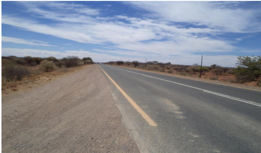
The N14 from Kathu toward Industrial road for entrance to the New Olifantshoek substation
