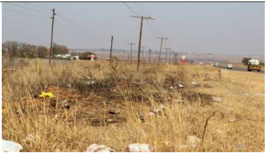
Figure 2: Eskom distribution line along the landfill side and the R537
