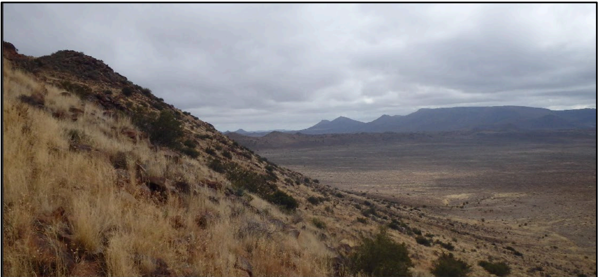
Contextual Images of the Development Area, showing the area of the proposed powerline route
