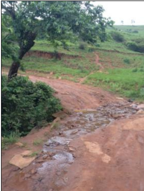
Photo 7: View of the fifth causeway site on the Mahlabathini Road.
