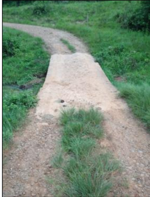
Photo 2: View of the proposed causeway site on the D1510 Road.
