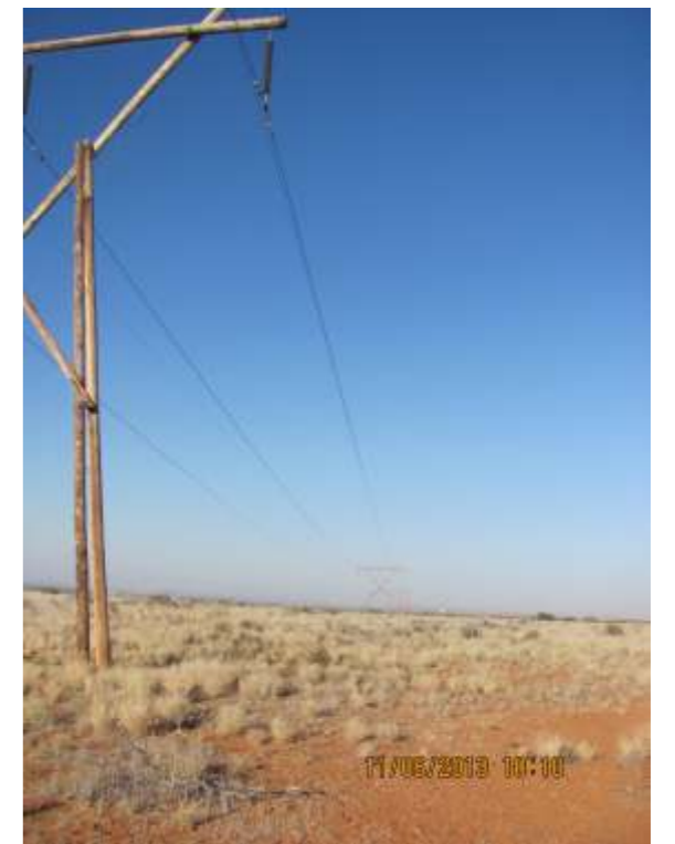
Figure 9: Existing 133Kv Powerline on the adjacent property.
