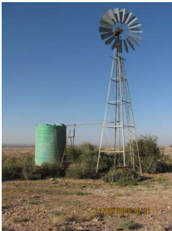
Figure 8: Showing existing borehole on site which is been investigated as a potential water source for the washing of panels.
