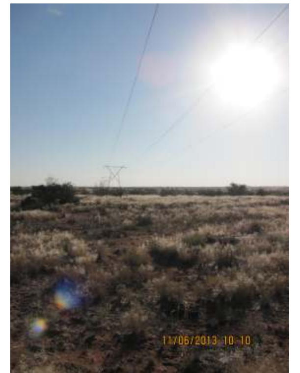
Figure 10: Existing 133Kv Powerline crossing the property.
