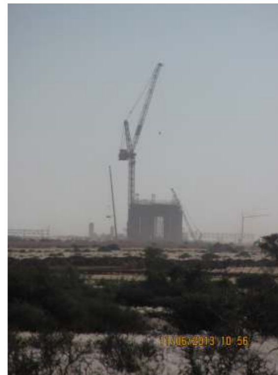
Figure 7: Showing Concentrated Solar Power Plant (CSP) currently under construction on an adjacent property.
