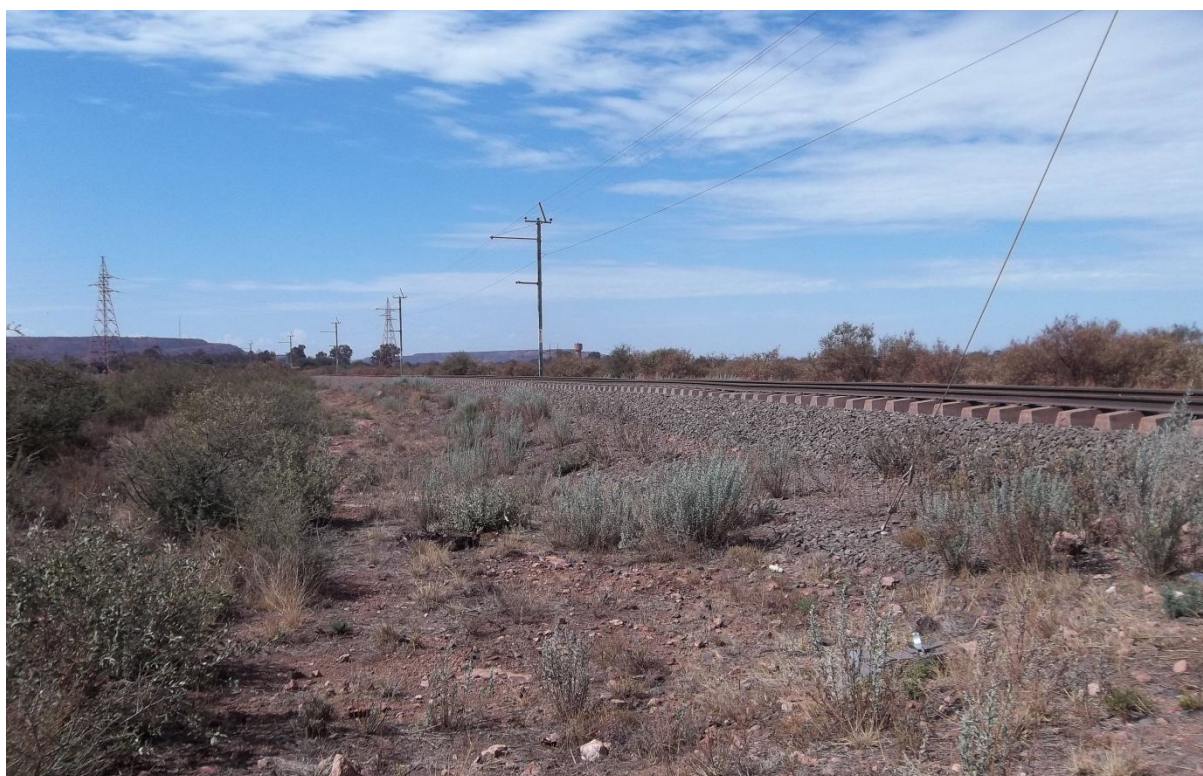
Plate 6: View towards the south . Photo taken at the point where the existing 275 kV power line crosses the old Postmasburg – Hotazel railway line.
