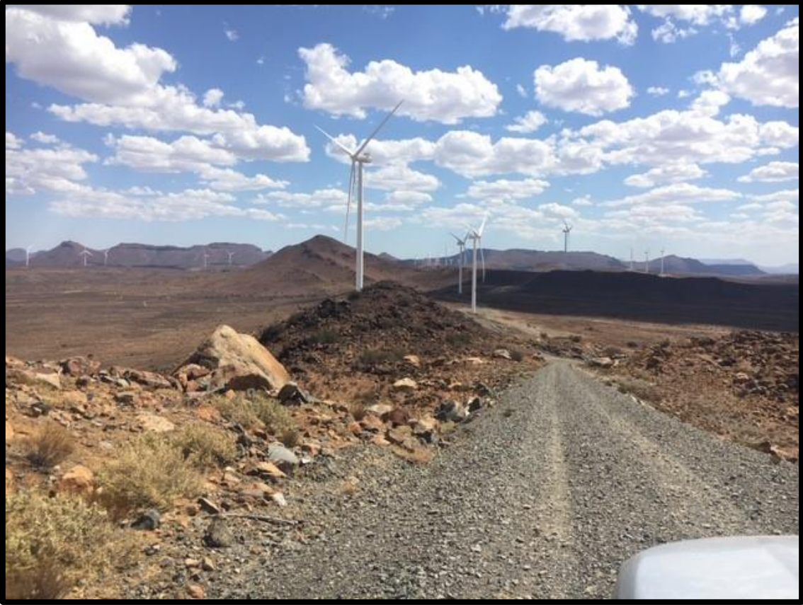
Images of the existing Noblesfontein service roads.
