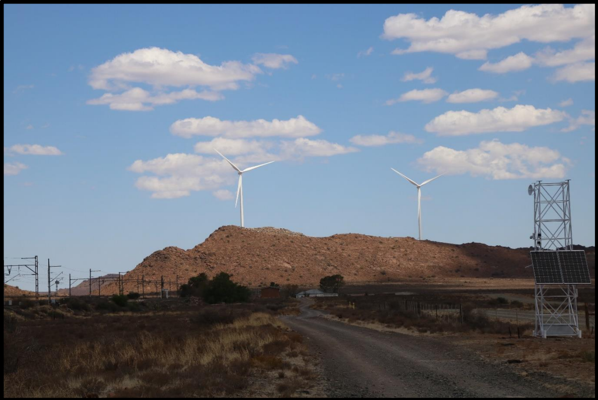
Various views of the existing Noblesfontein turbines.
