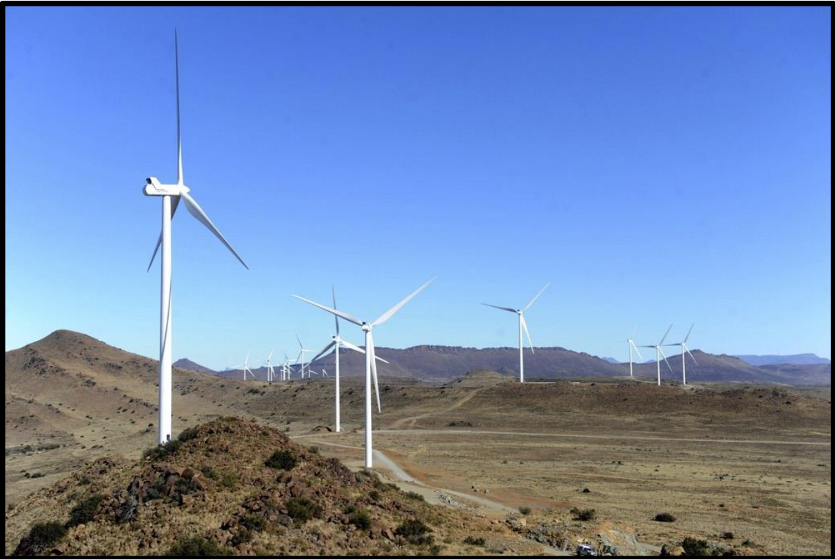
Various views of the existing Noblesfontein turbines.
