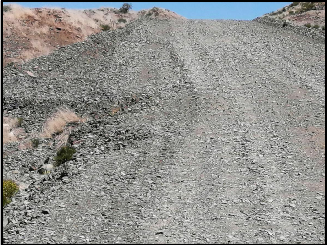
Images of the existing Noblesfontein service roads.
