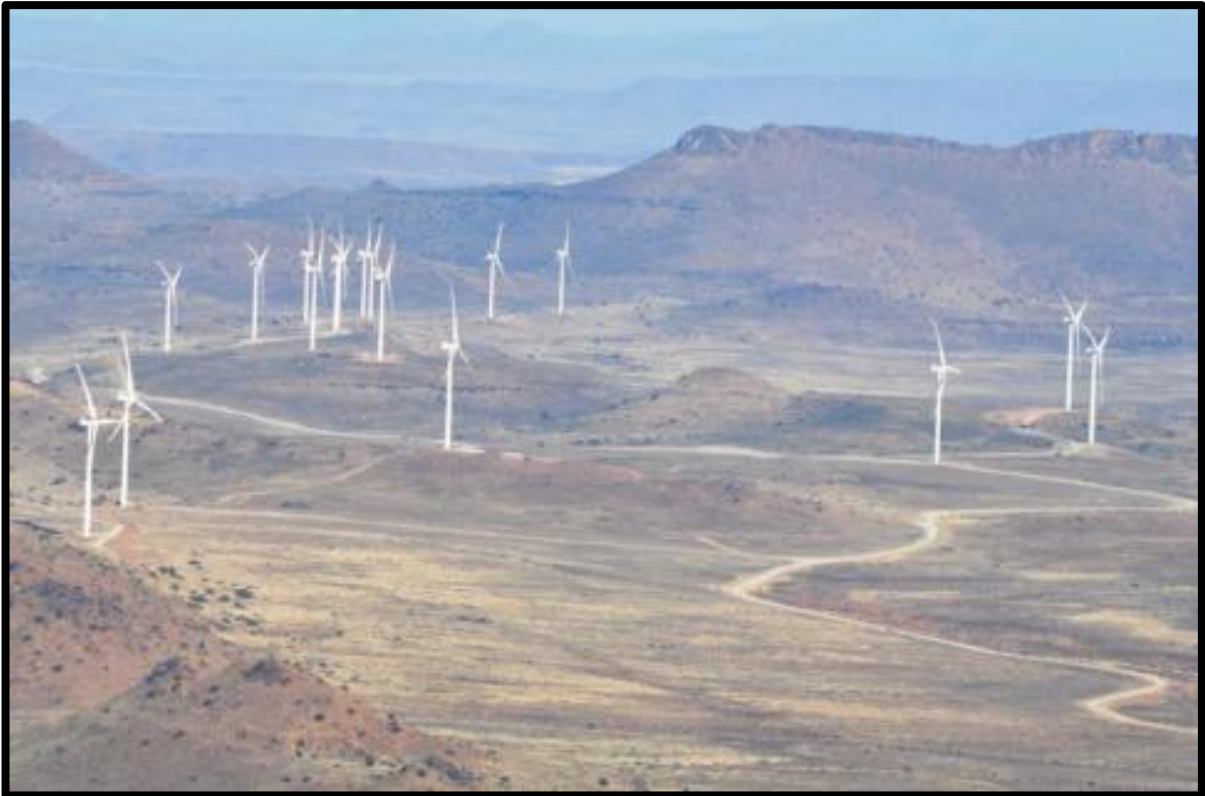
Various views of the existing Noblesfontein turbines.
