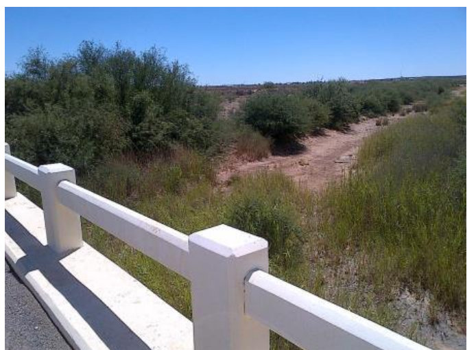
Photo 18: View from bridge over Sak River looking north-west
