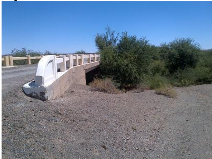
Photo 17: Sak River bridge crossing. Pipeline will be attached to the bridge
