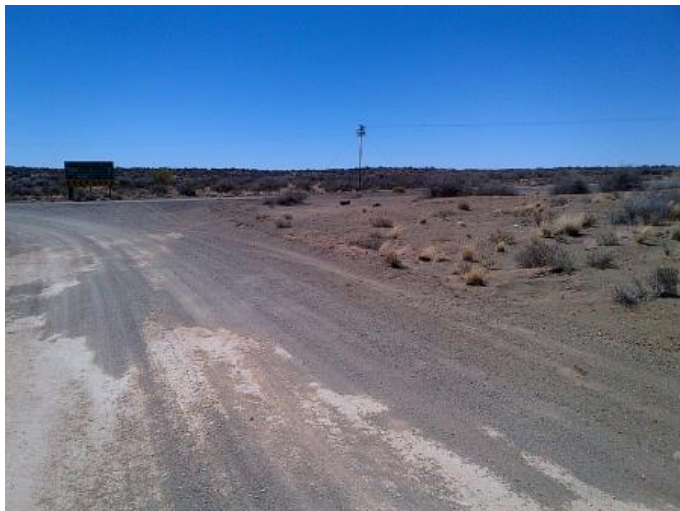
Photo 15: Intersection of R353 and R357
