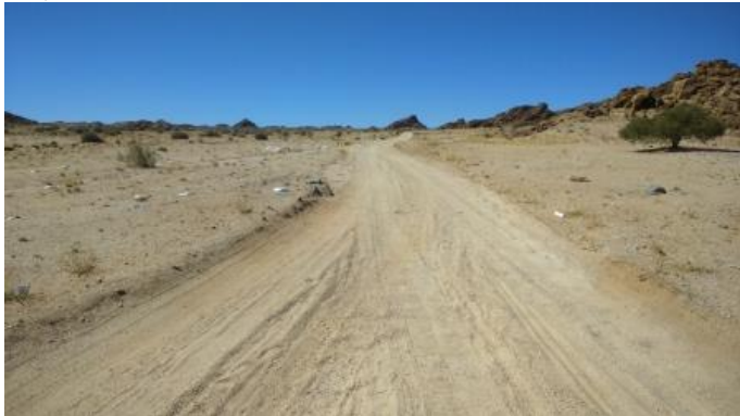
Photo 15: Taken from point 4, looking south down the pipeline and overhead electrical line route (between the pumpstation and SPV site)
