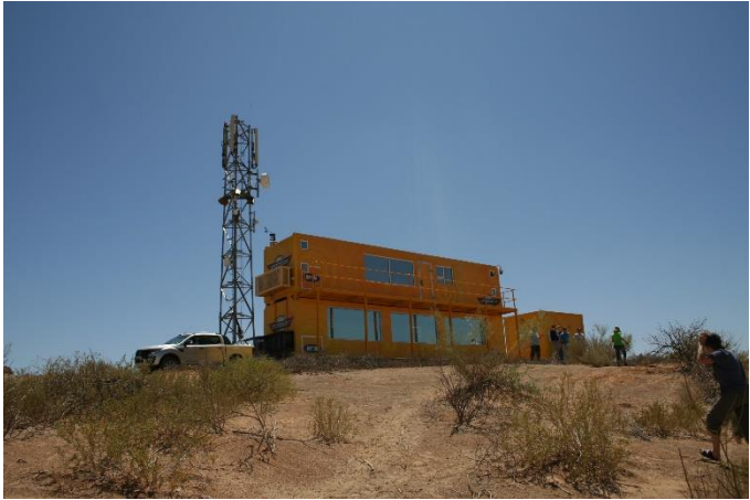
Photo 8: The existing control tower housed in modified shipping containers located at the Speedweek/landside camp. Taken at Point 7
