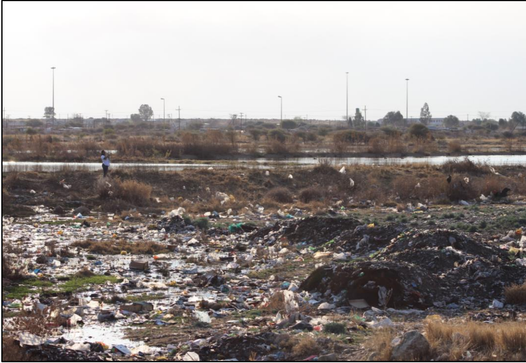
Figure 17: View west towards the oxidation pond. Note the effluent from the pond within the waste
