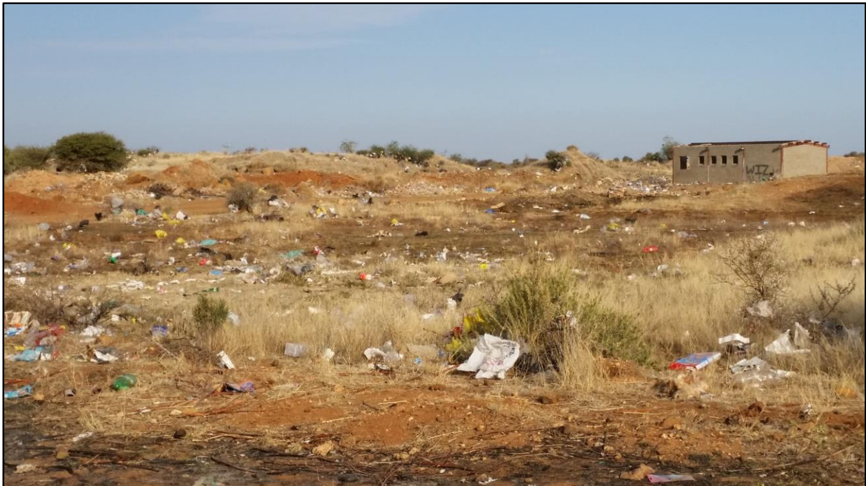
Figure 6: View towards the south south west showing the dilapidated structure on site
