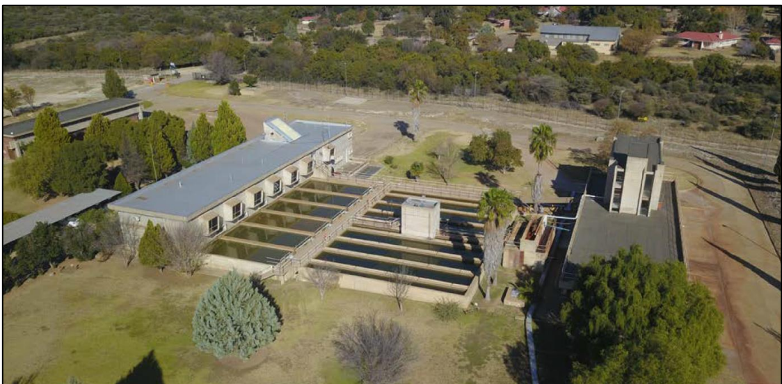
Figure 3: View of Delportshoop Water Treatment Works
