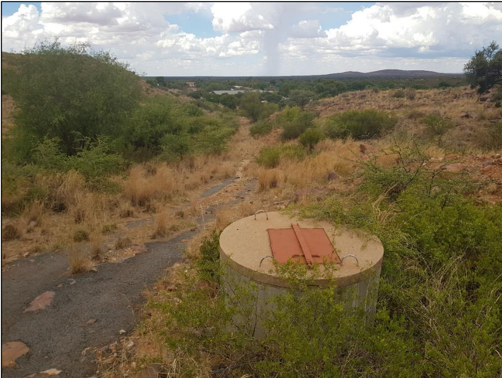
Figure 14: Views along pipeline from Gloucester to Olifantshoek Reservoir
