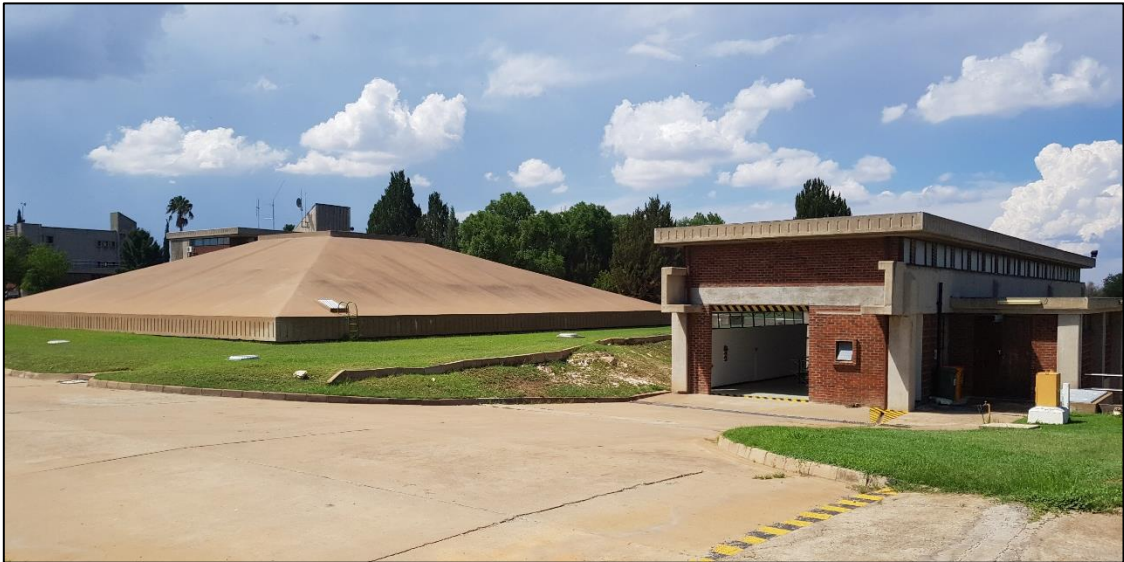
Figure 2: View of Delportshoop Reservoir and Pump Station
