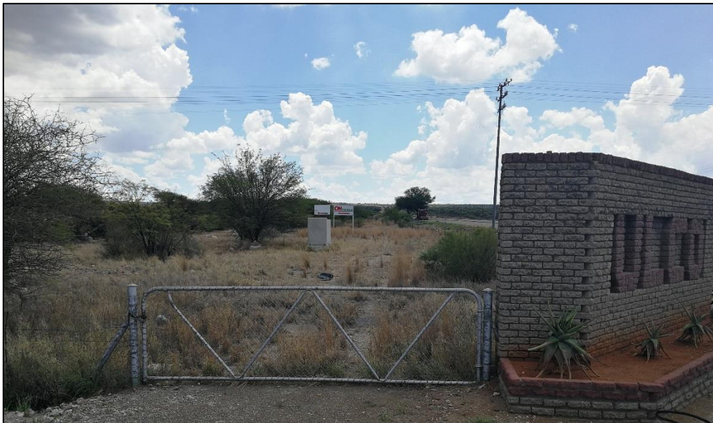
Figure 4: Views of pipeline from Delportshoop to Kneukel Pump Station
