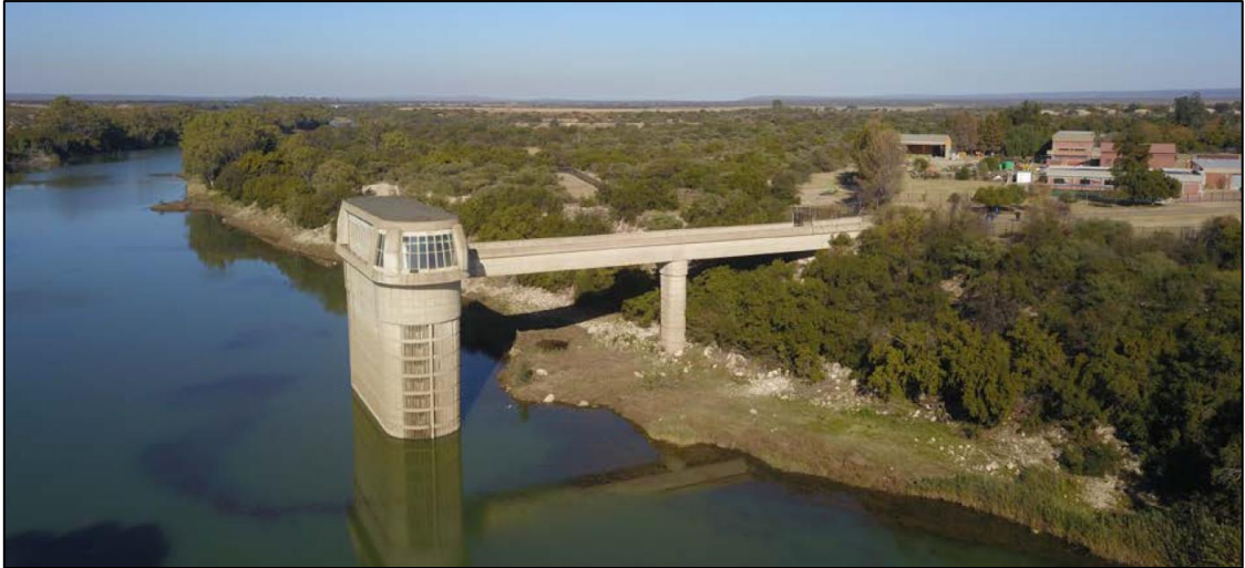
Figure 1: View of Delportshoop Abstraction Works on Vaal River
