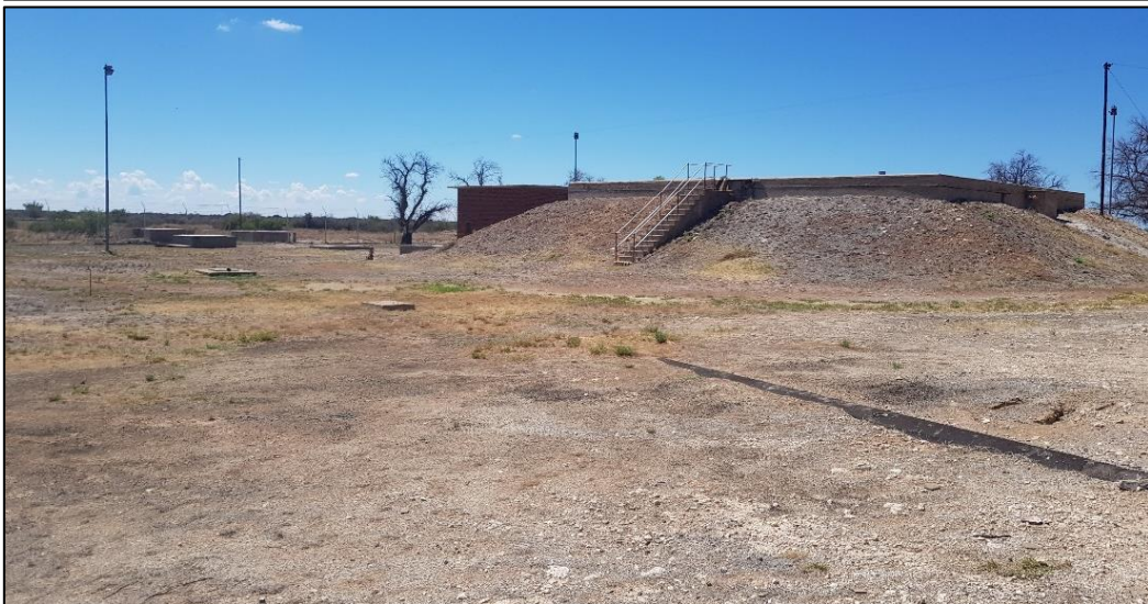
Figure 7: Views of Trewill Pump Station and Sump
