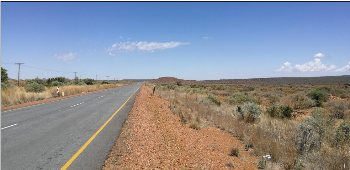
Figure 11: Views along pipeline from Clifton Reservoirs to Postmasburg
