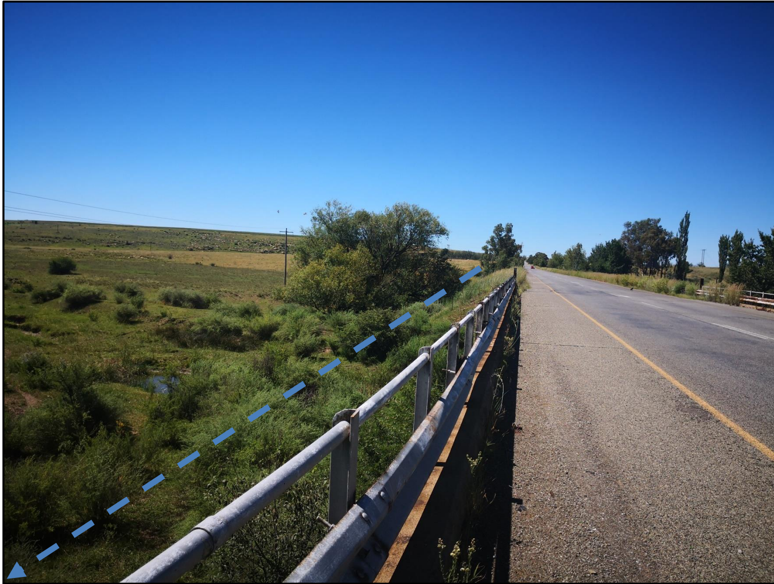
Photo 9: Route along R707, estimating where the pipeline runs
