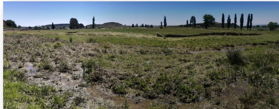
Photo 4: Stormwater outlet to be crossed by the pipeline
