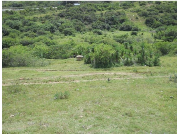
Manhole along sewage pipeline servitude (facing north) with the R72 in the background.
