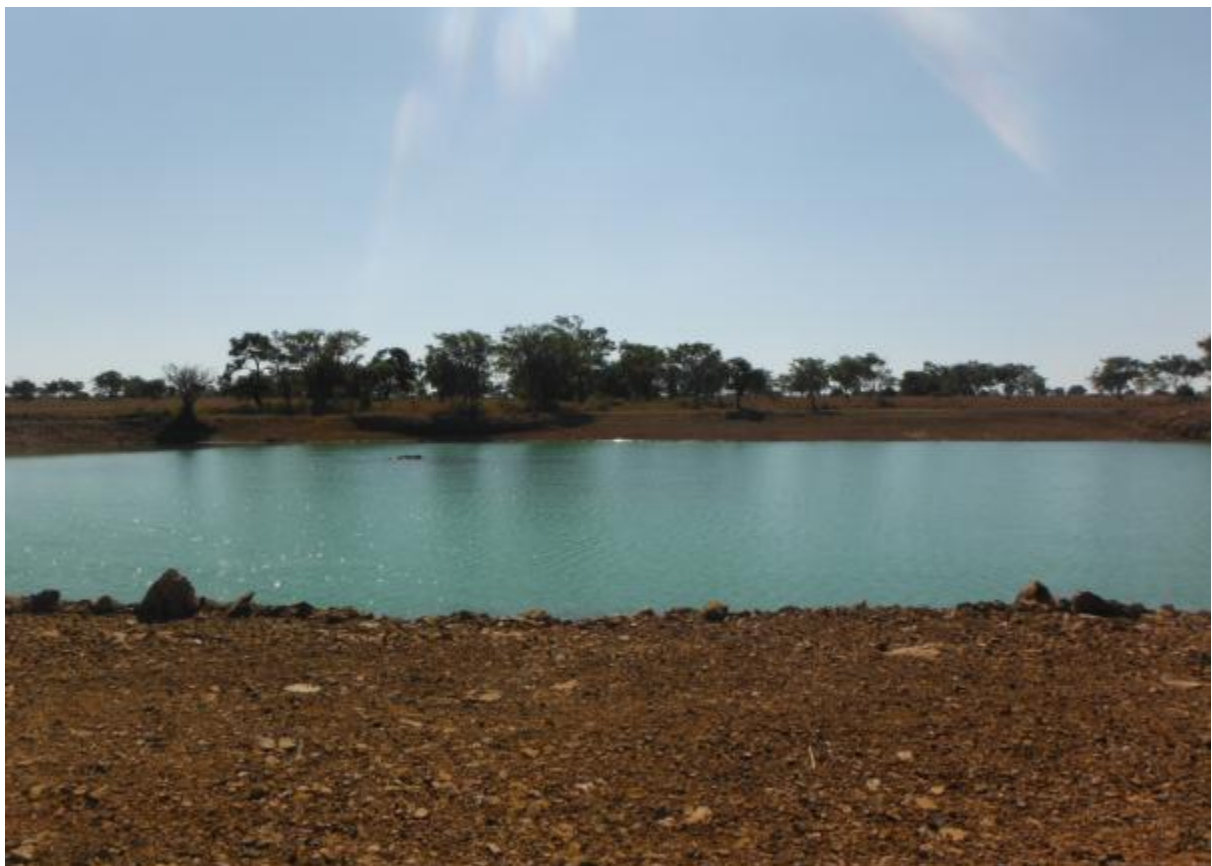
Picture 1: View of the western dam facing north
