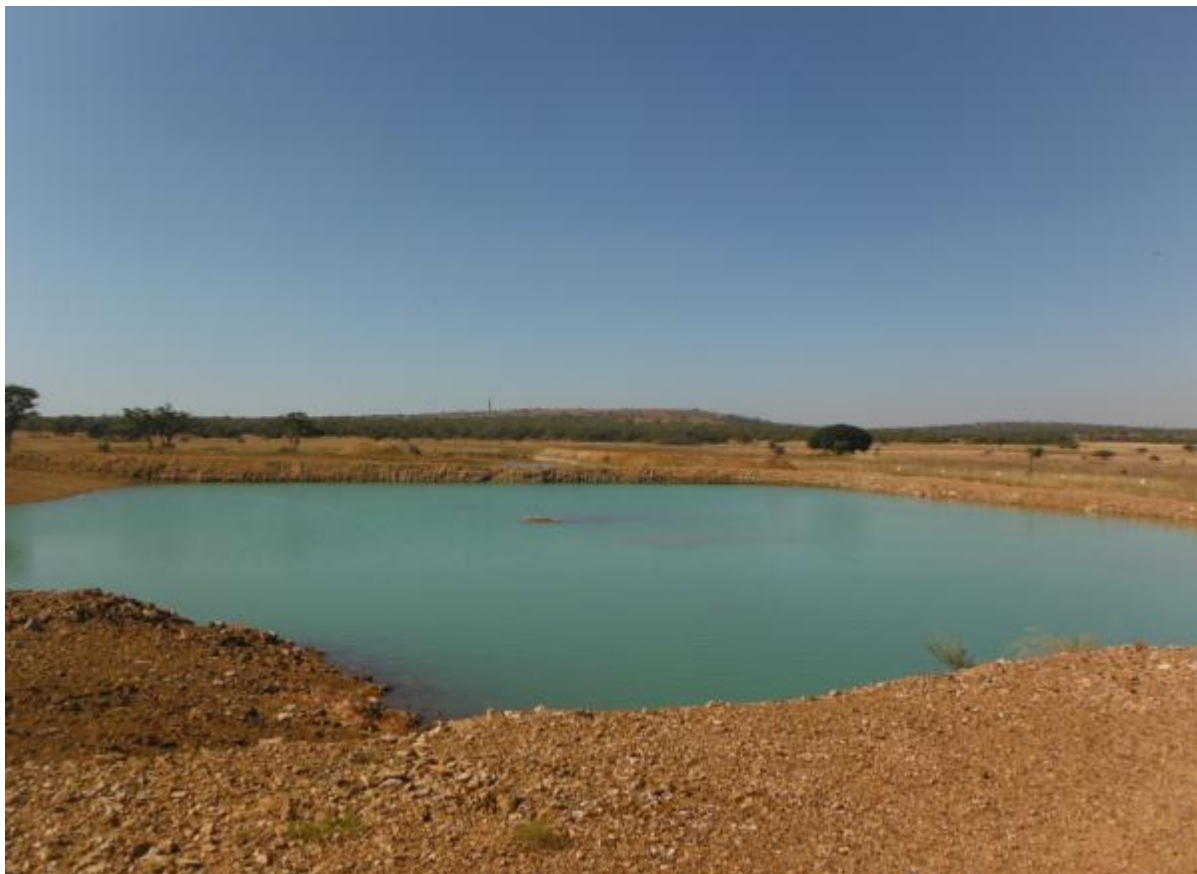
Picture 6: View of the western dam facing east
