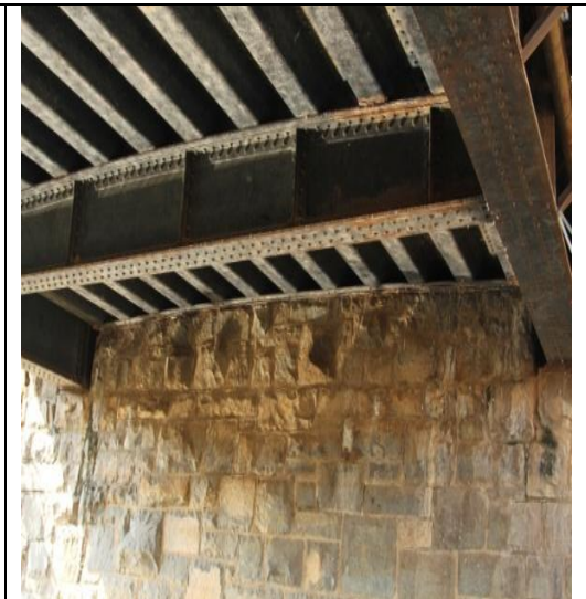
Existing Conrad Bridge viewed from beneath
