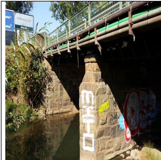
Existing Bridge to be expanded
