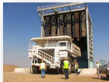
Typical opencast tipping and crushing facilities
