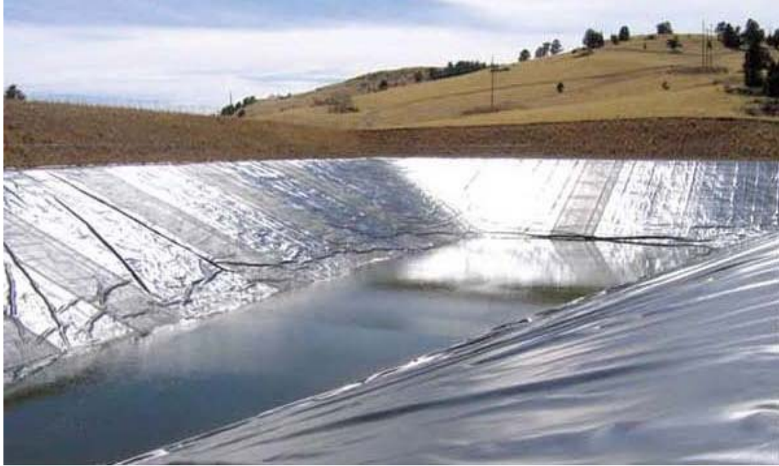
Figure 17: Typical Lined Dam (DWAFA4, Aug 2007)
