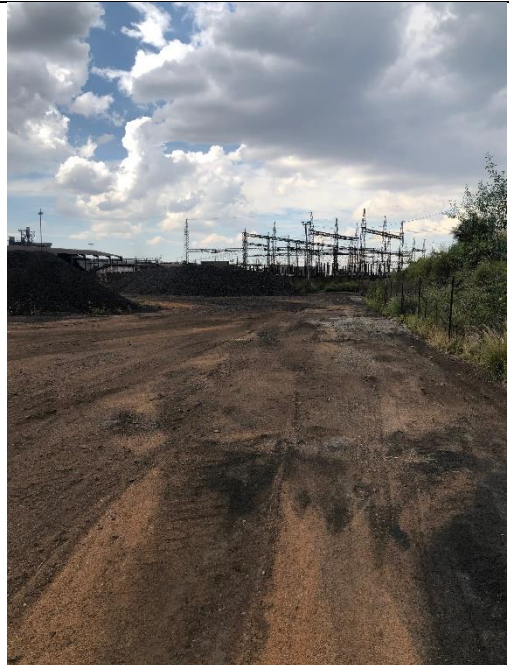
View from site looking north east towards Eskom HT yard (stockpiles visible)
