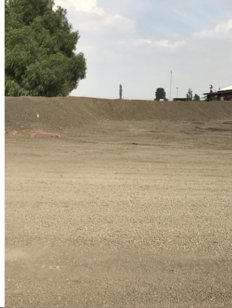
Looking south towards building (offices) and TMR plant
