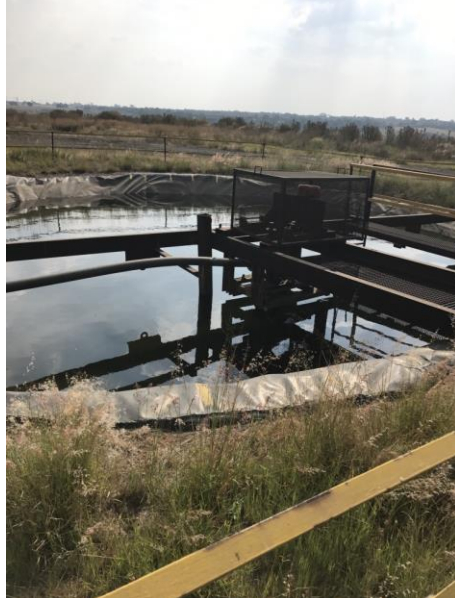
PCD for Fe-Cr slimes dam with pump for treatment and reuse
