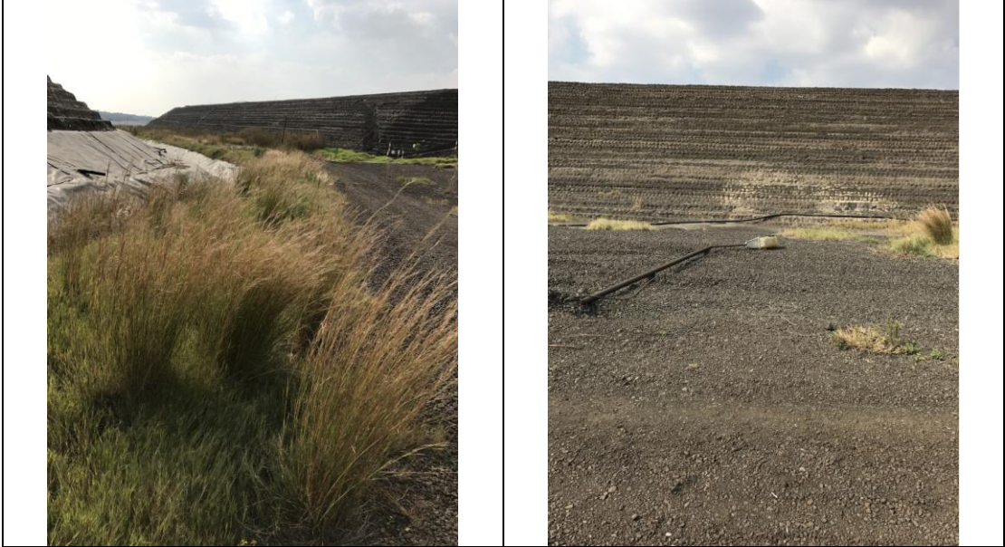
Looking east towards the Mn Slimes dam
