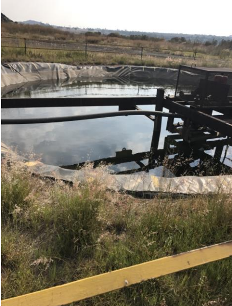
PCD for Fe-Cr slimes dam with pump for treatment and reuse
