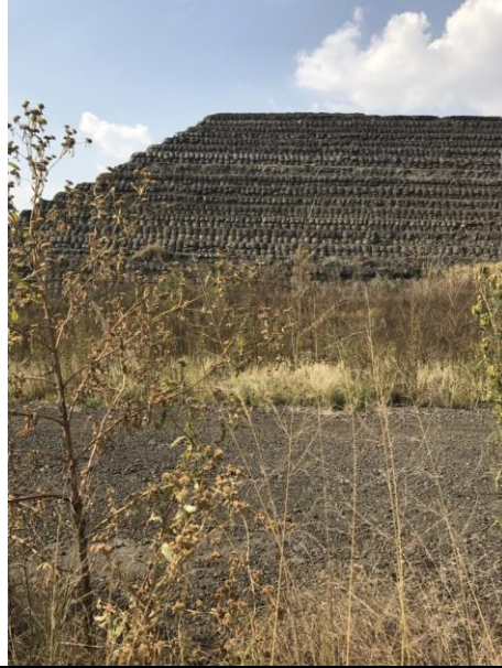
View of Fe-Cr Slimes Dam from north
