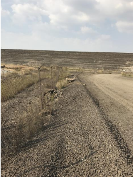
Looking east along Fe-Cr slimes WDF and towards Mn slimes dam
