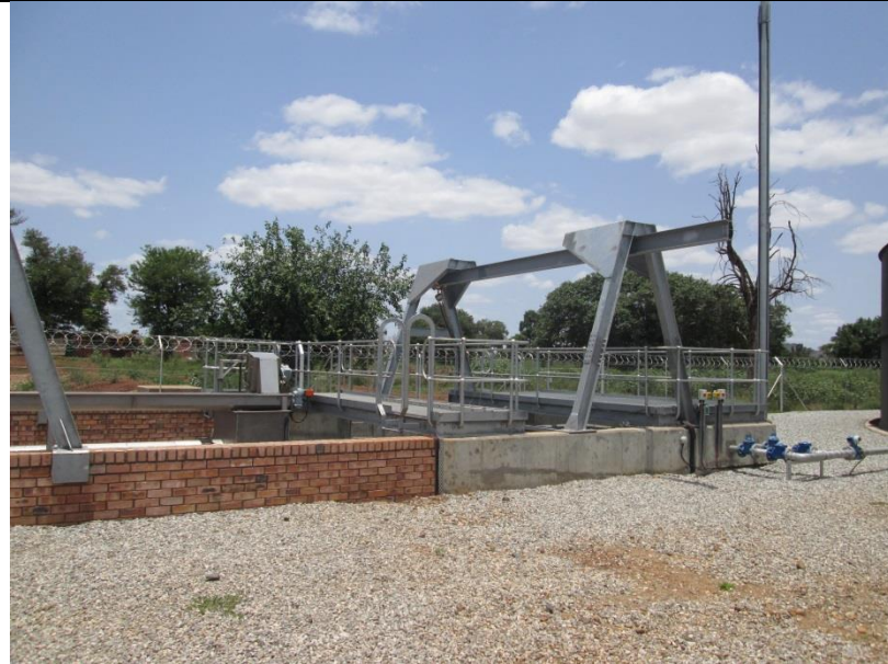
Photo 2: View of the existing package plant inlet works
