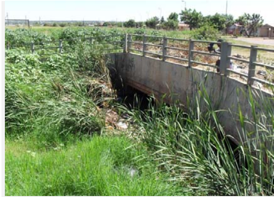
Figure 2: Stormwater infrastructure on the boundary of the southern site
