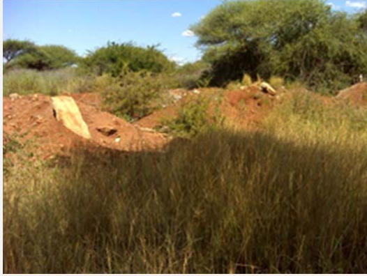
Figure 5: Earthworks and dumping
