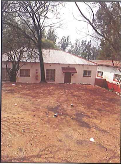
North: Facing the northern boundary and permanent accommodation on site
