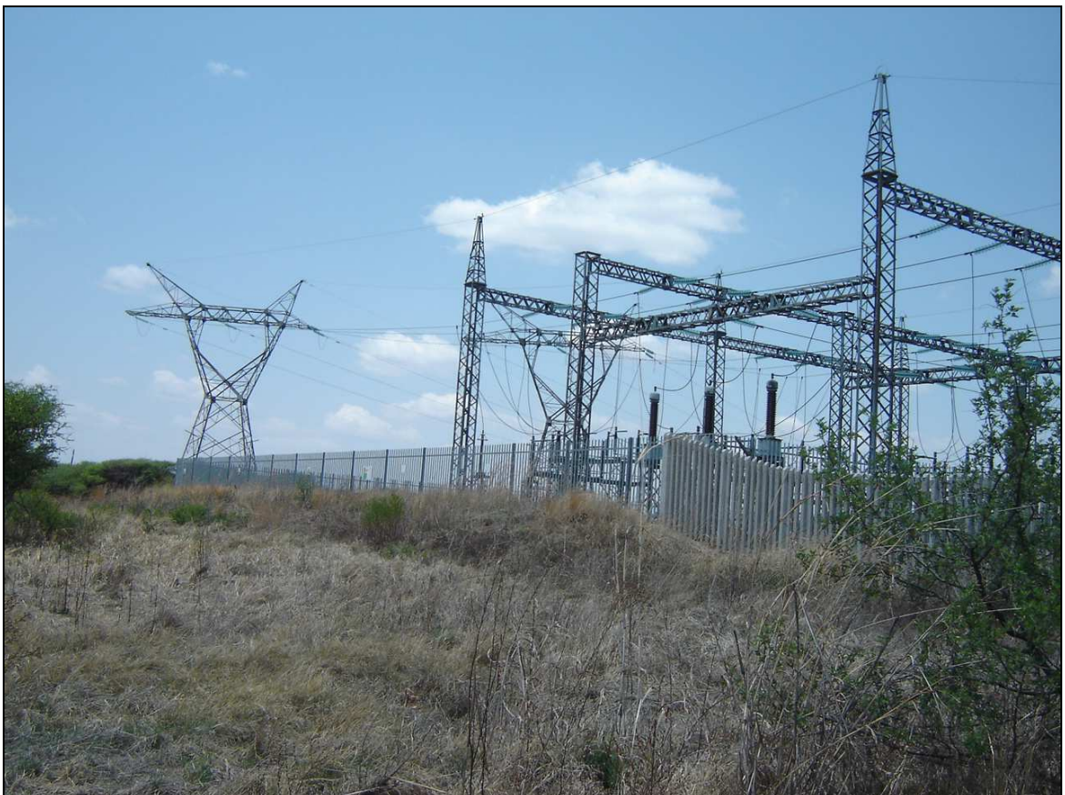
Figure 4: View from the site to south-east
