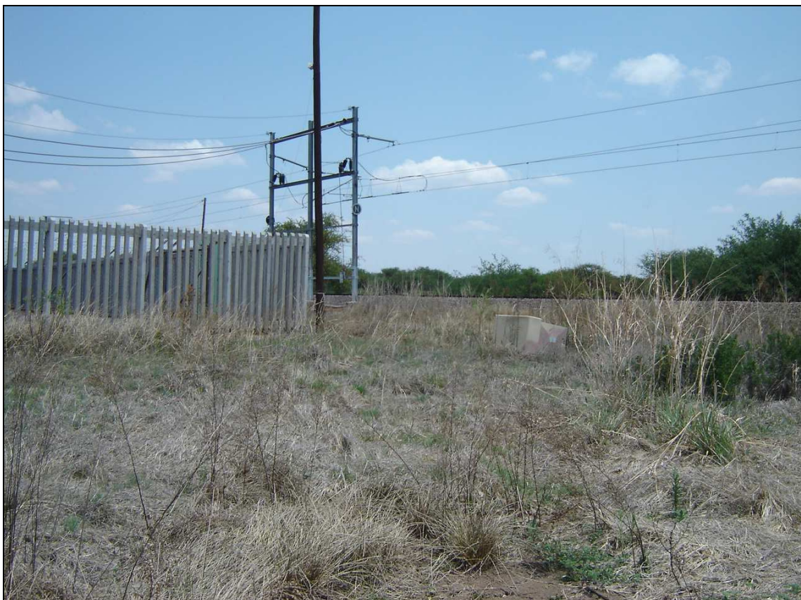
Figure 6: View from the site to south-west
