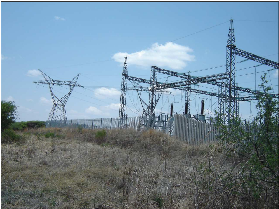
Figure 4: View from the site to south-east
