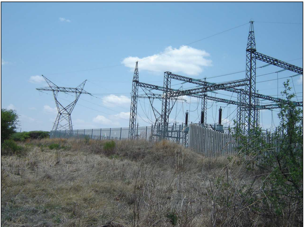
Figure 4: View from the site to south-east
