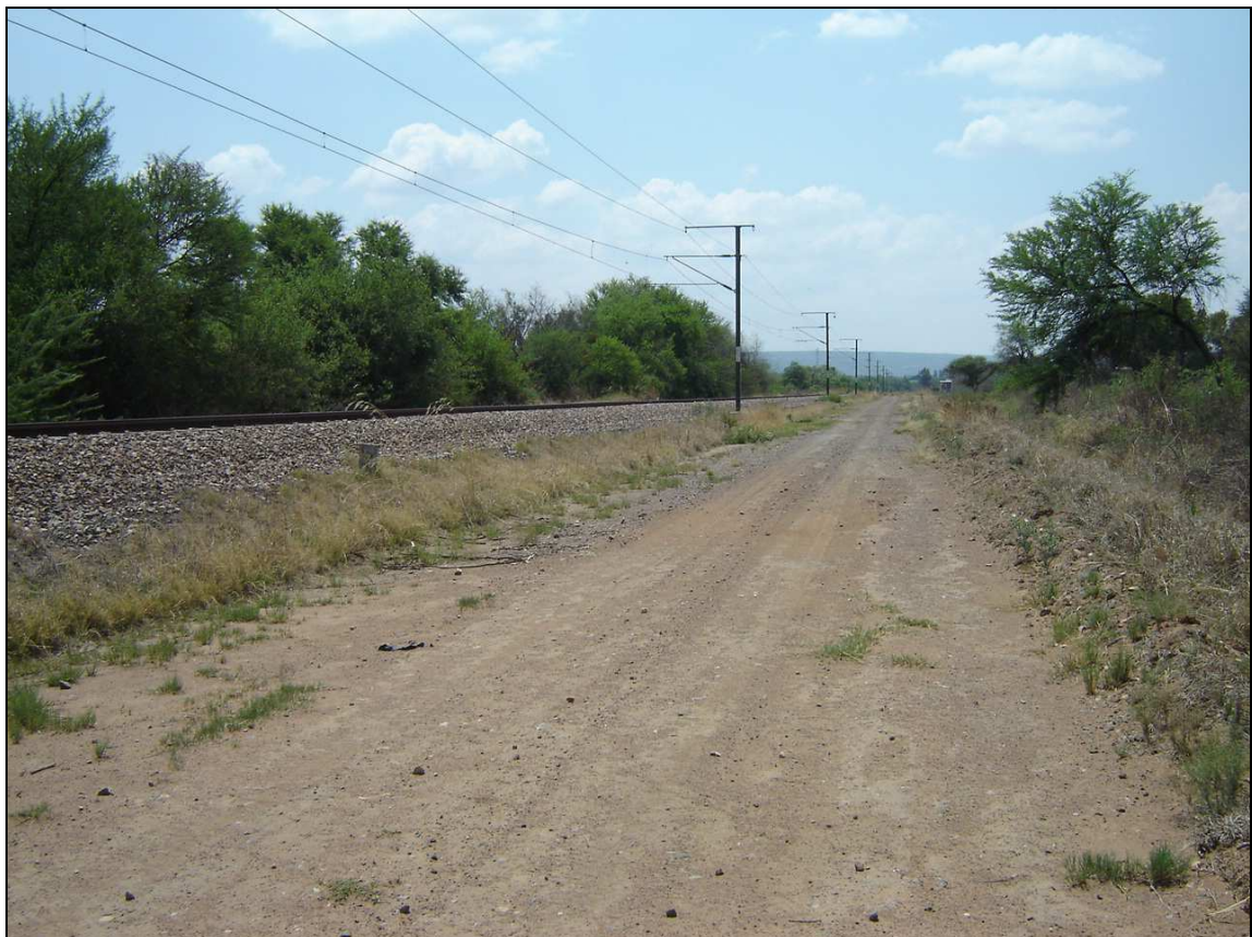
Figure 10: View of access road
