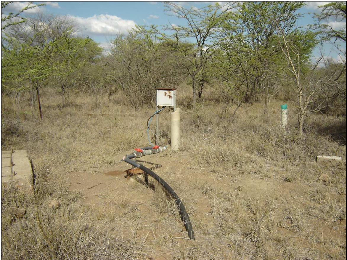
Figure 9: Existing borehole on site
