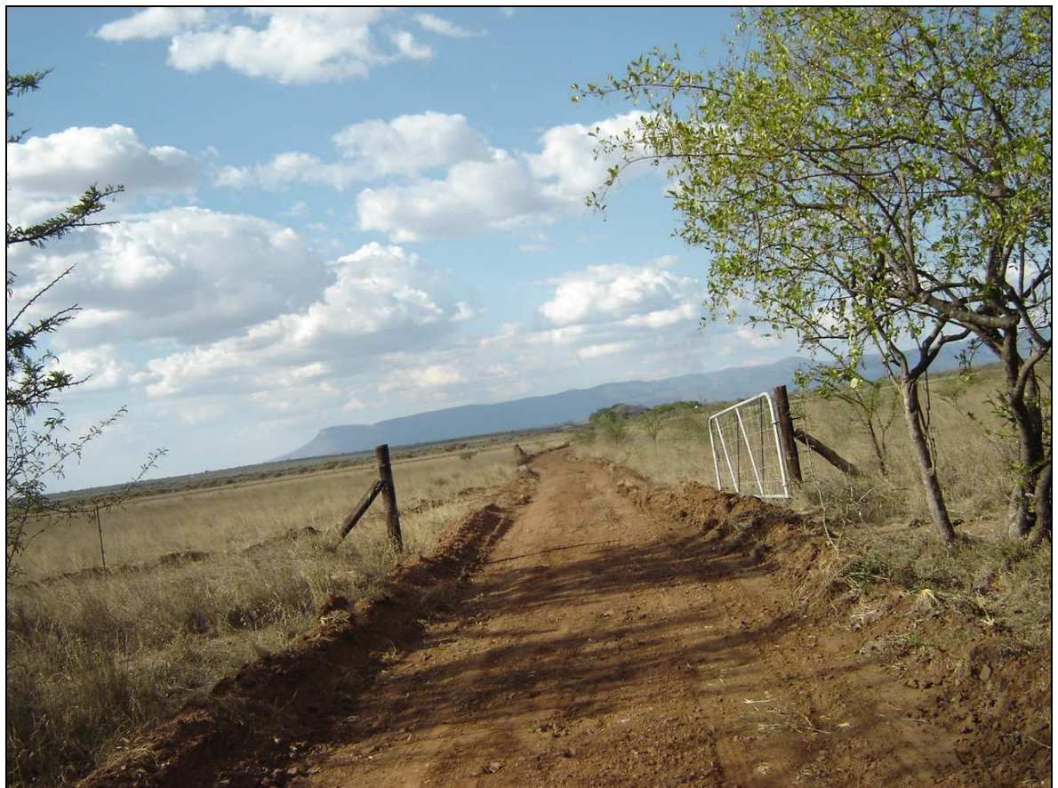
Figure 12: Existing road on site
