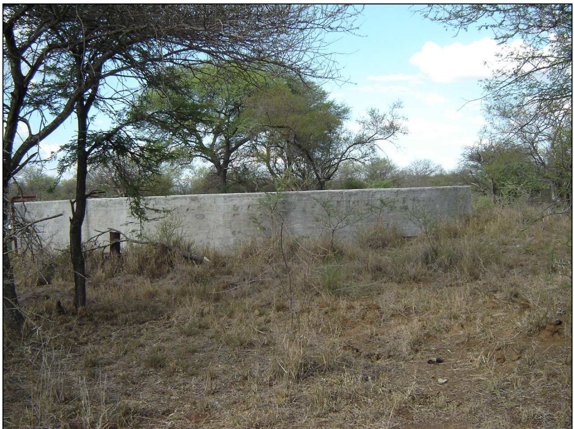
Figure 10: Existing concrete dam on site
