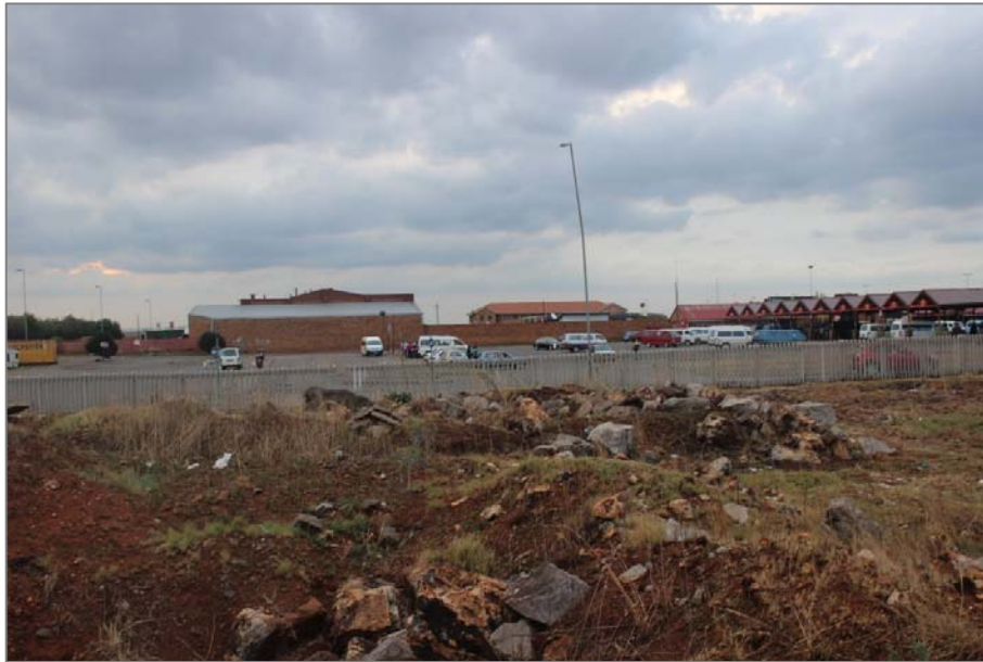
Figure 7: View West of the site which displays the concrete palisade perimeter fence surrounding the Vosloorus Taxi Rank (background)
