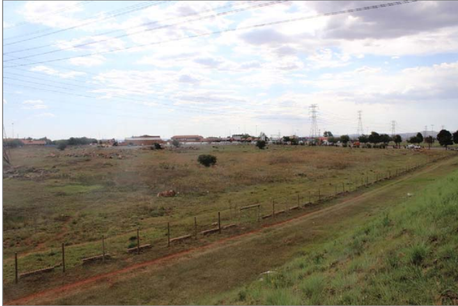
Figure 9: Perimeter fence which runs parallel to the N3 highway
