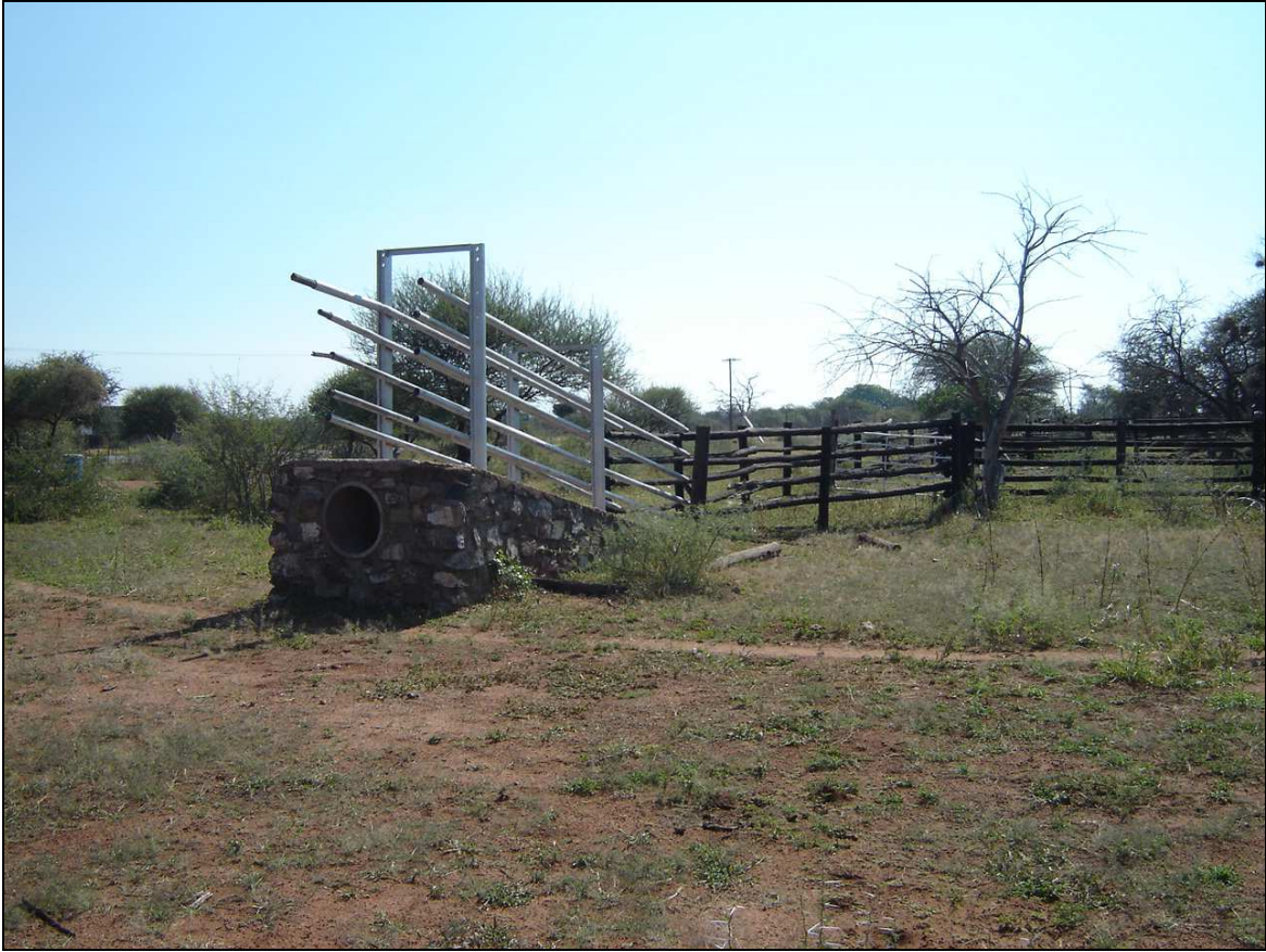
Figure 1: View from the site to the north
