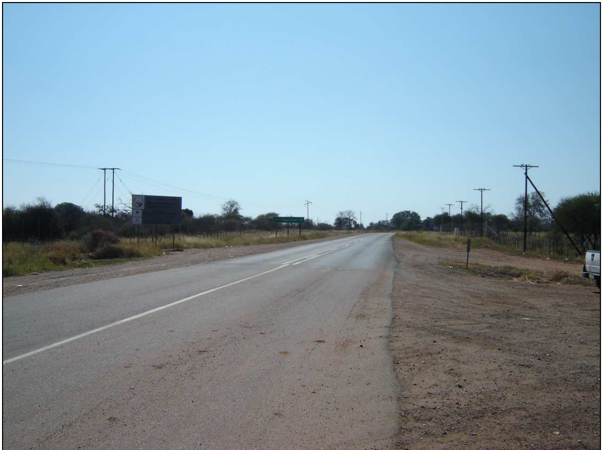
Figure 10: View of access road R572
