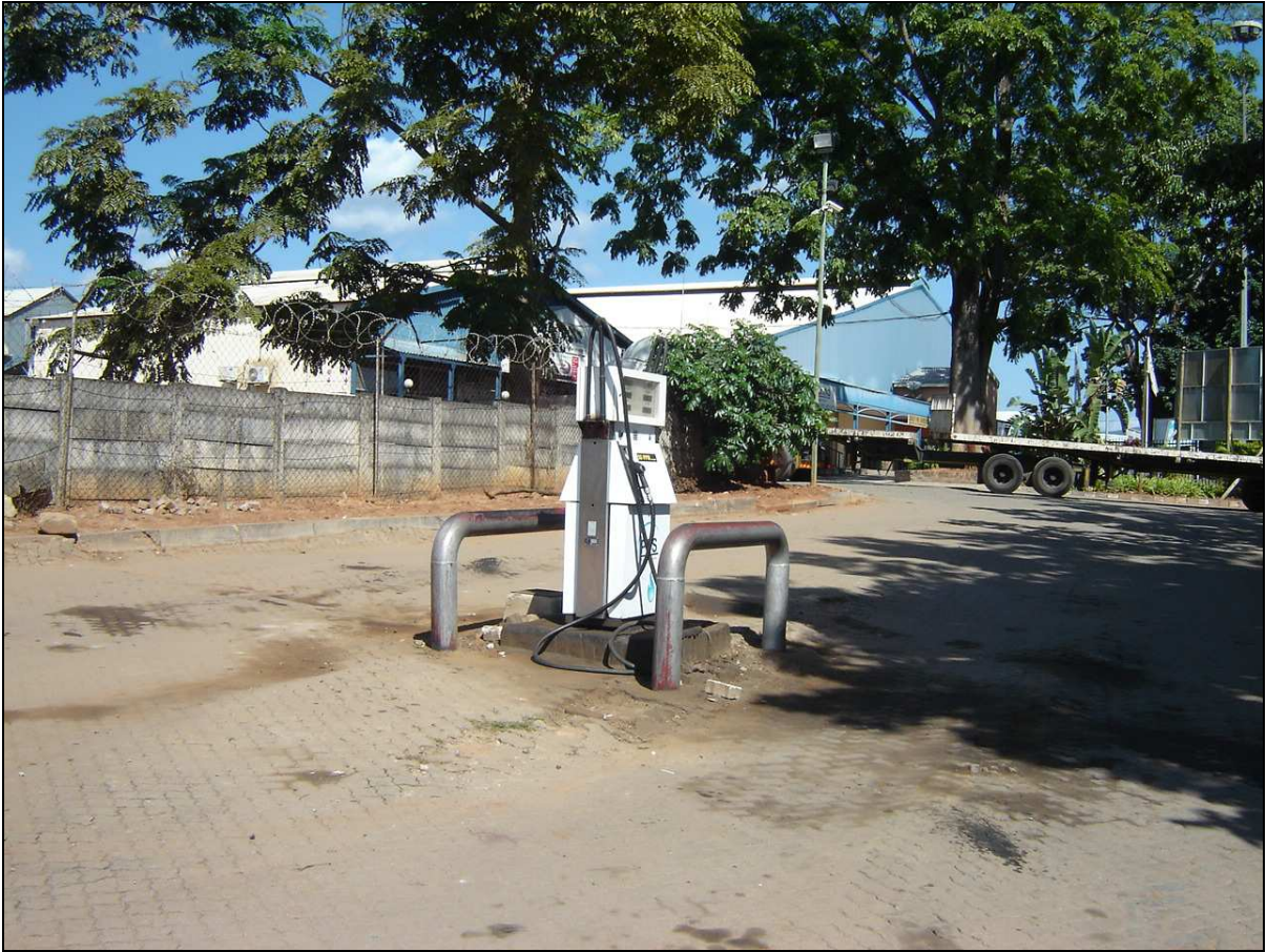
Figure 11: Existing pump on site
