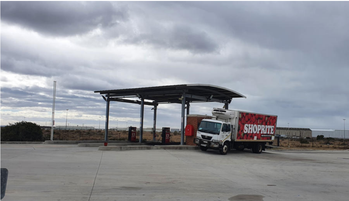
Photo 4: Existing fuel depot.
