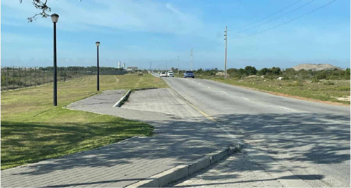
Photo 23: Public Transport Embayment adjacent to the Existing Shoprite Entrance on the R102. Photo credit GPL Consulting.
