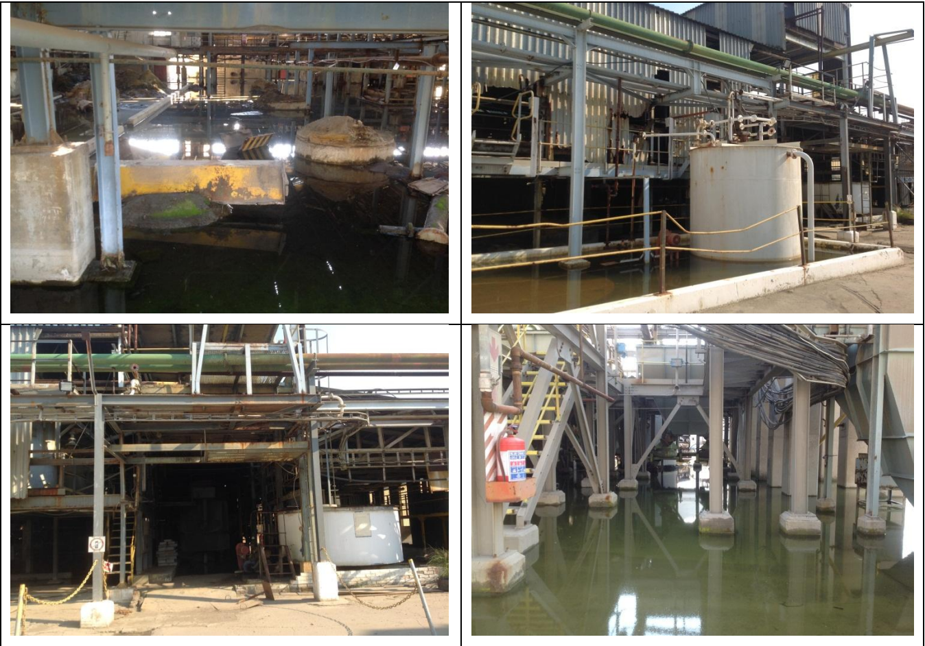
2 – Filtration Plant Area: Looking in a Easterly direction from the centre of the site being demolished.
