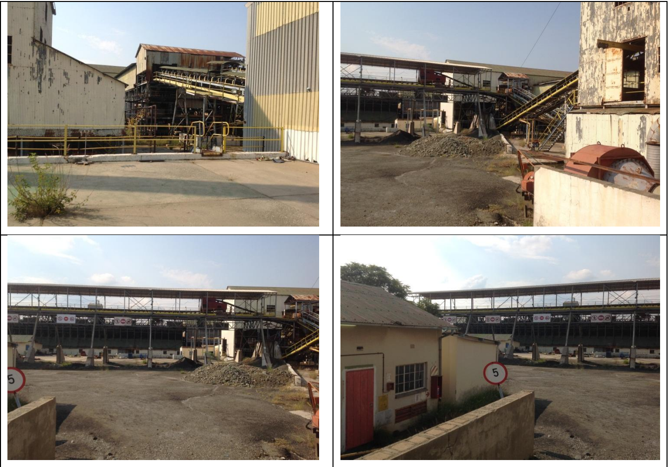
6 – Crusher Plant Area: Looking in a Southerly direction from the centre of the site being demolished.
