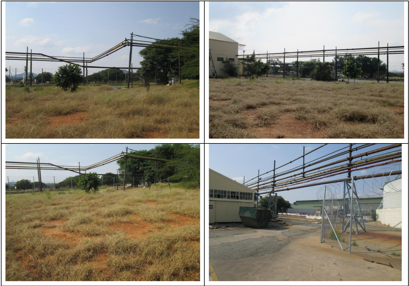
8 – Redundant Pipe Line Infrastructure: Looking in a North Westerly direction from the centre of the site being demolished
